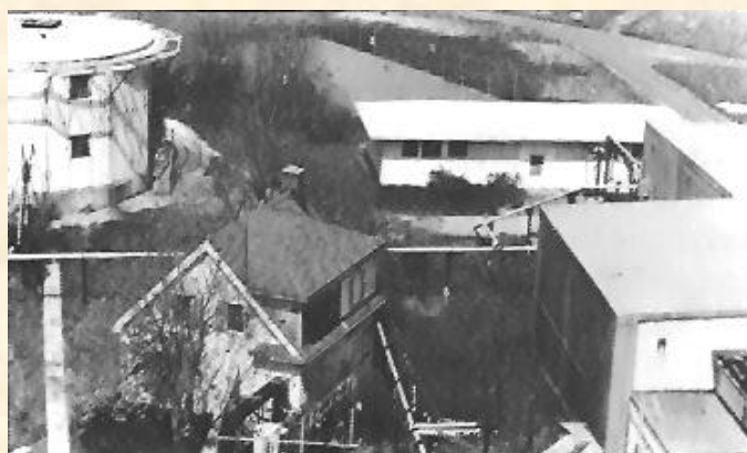
Montauk Air Force Base An overview looking north. The computer control center is to the right. Just behind that is an office building. The round building to the left is a radar building that was also used for storage
