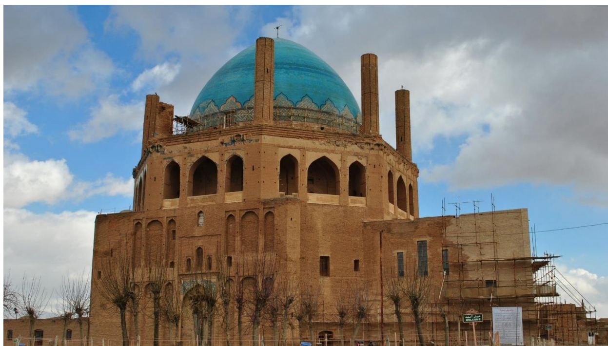
Figure 1: The Soltaniyeh dome as seen in 2011 after modern reconstruction efforts on the dome. Repairs are ongoing on restoring other features of the dome, such as the minarets which were heavily damaged and eroded.
