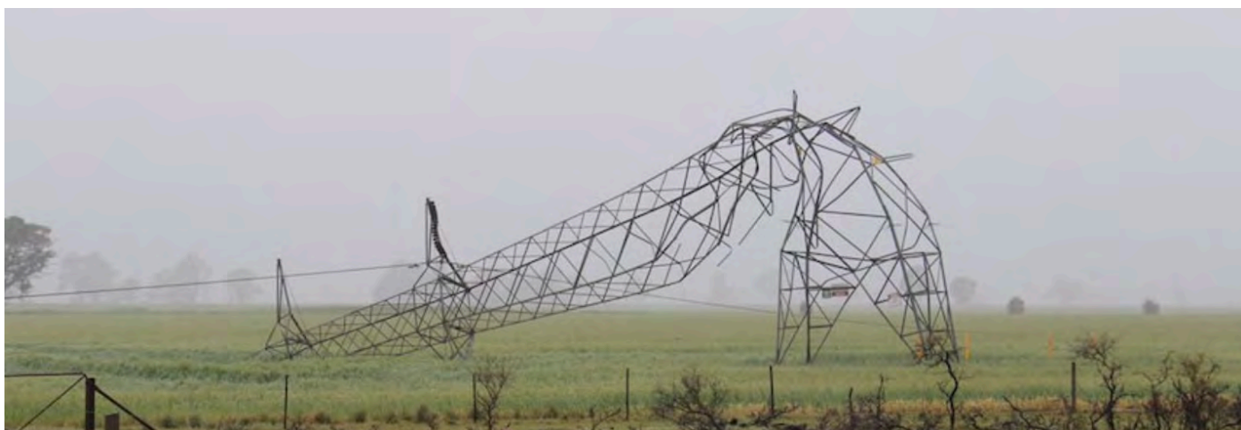
Photo - A collapsed electricity pylon near Melrose, South Australia in 2016 (ABC News, 2016).
