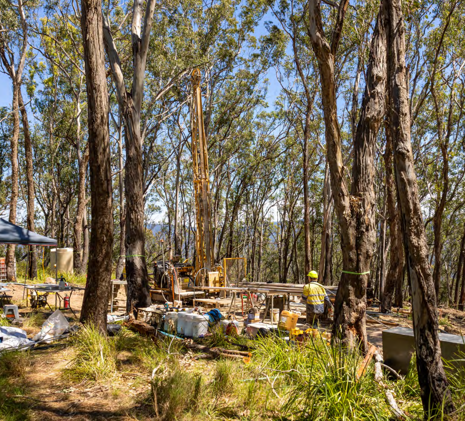
Photo - Geotechnical investigations near the project's upper reservoir.
