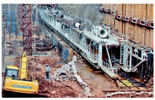
On 8th July, 2013, a 96 metre long completely assembled underground Tunnel Boring Machine began tunneling between Jama Masjid and Delhi Gate Metro stations. This is the longest TBM that has ever been used in Delhi Metro project and weighs approx. 500 tons.
