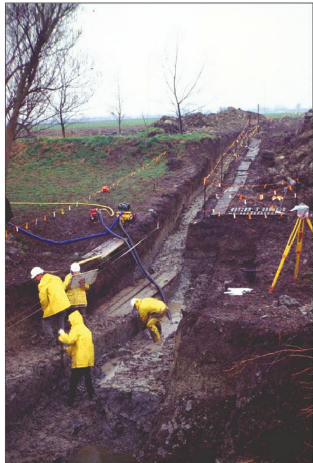
Plate 2.2 Excavation of the Old Tillage, Waterbeach (1993) in progress
