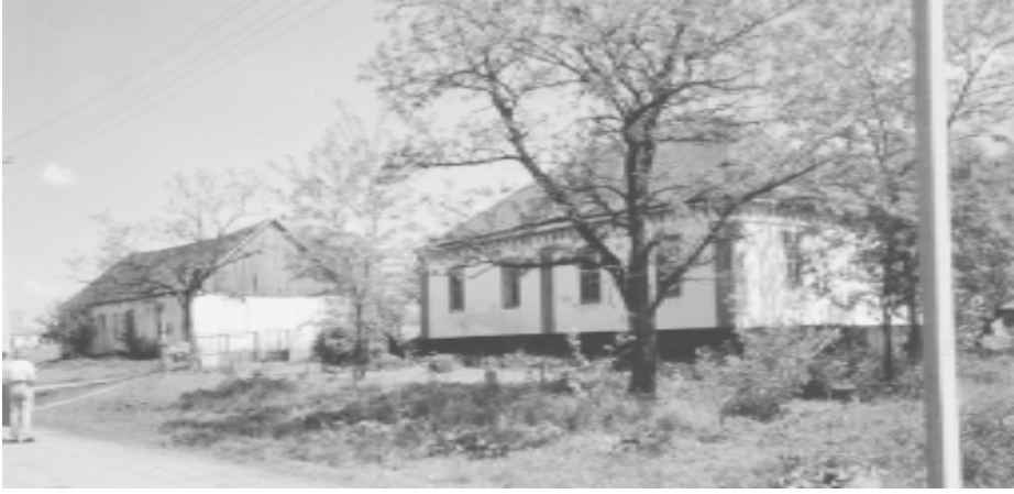
The former village school and worship house in the village of Heuboden, home of KG delegate David Klassen (1813-1900), who later settled in Rosenhof, Manitoba. The buildings probably date to the 1890s.
