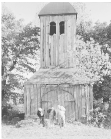
An abandoned windmill at Neunhuben, the place of residence of KG founder Klaas Reimer (1770-1837) after he married Maria Epp, daughter of the esteemed Danzig Aeltester Peter Epp. The building is now used as a storage house for the adjacent cemetery--see also cover photo. Here Milton and Margaret Toews, and Gerald Wright inspect the writing in a concrete pad poured by the front door.
