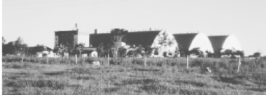
Wheat silos and flour mill at Camp 9 Sommerfeld Colony.
