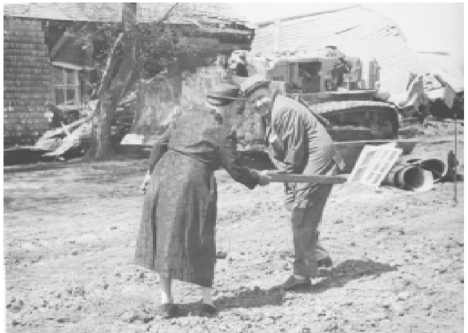
1960 The "G. G. Kornelsen housebarn" being torn down by a developer to make room for a commercial development. In the photo the developer A. D. Penner receives a mock spanking from his mother for being so naughty. Photo courtesy of Steinbach: Is there any place like it? (Steinbach, Manitoba, 1991), page 192. According to writer/historian Gerald Wright "the destruction of the buildings helped shock local preservationists into taking action that led to the establishment of Steinbach's new $4 million Mennonite Heritage Museum." Mr. Penner evidently did not much favour preservation of local culture and heritage and at one point boasted that "I have not spoken Low German now for years"--
