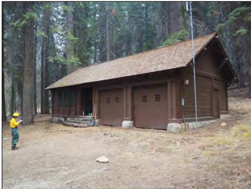
Photo 10 Cabin Creek Dormitory. View looking southwest.
