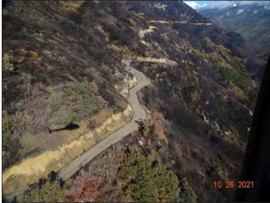
Photo 13 Mineral King Road. View looking northwest from helicopter.
