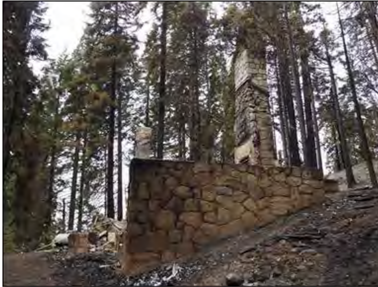
Photo 1 Redwood Mountain Ranger Station masonry remnants. View looking west.
