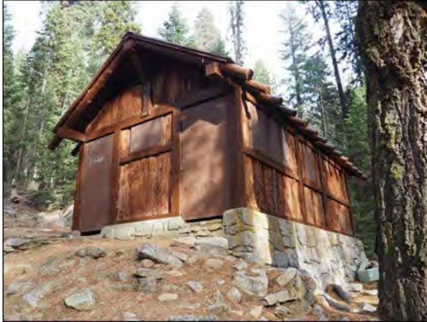
Photo 8 Lost Grove Comfort Station. View looking upslope, east.
