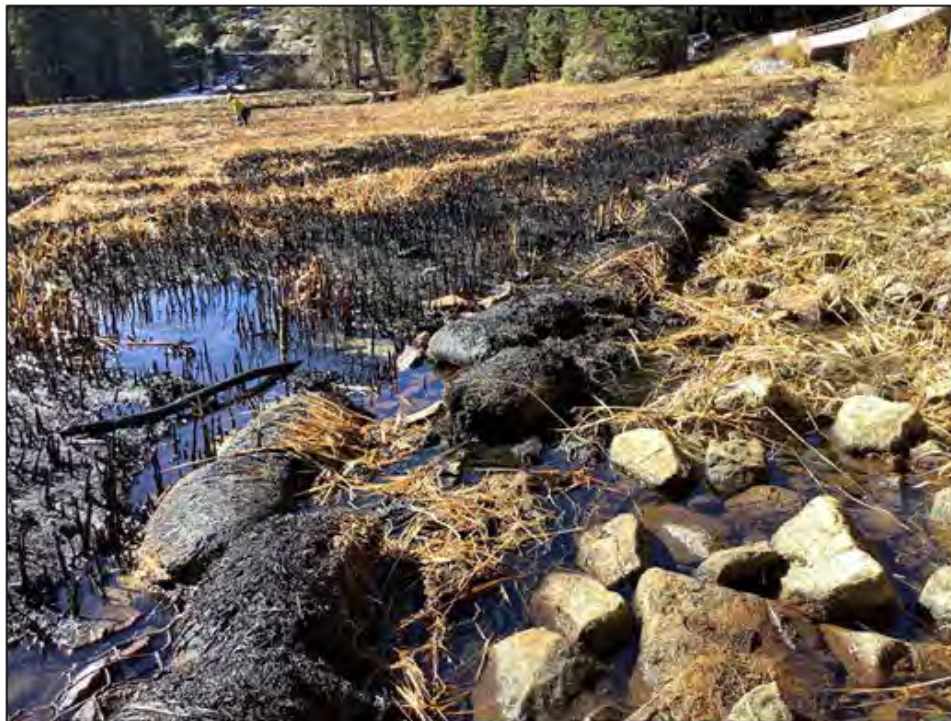
Figure 6. A row of sandbags designed to spread out surface flow in restored Halstead Meadow was damaged in the KNP Complex and started to fail in the October 25 storm.
