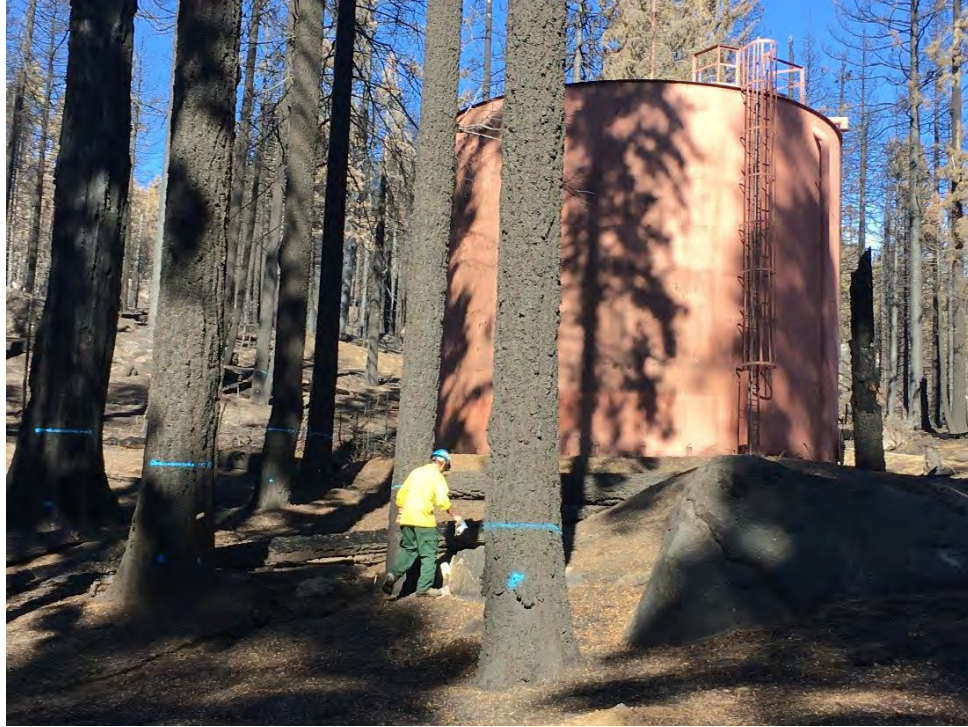
Matt Kennedy, Red Fir Effluent Tanks
