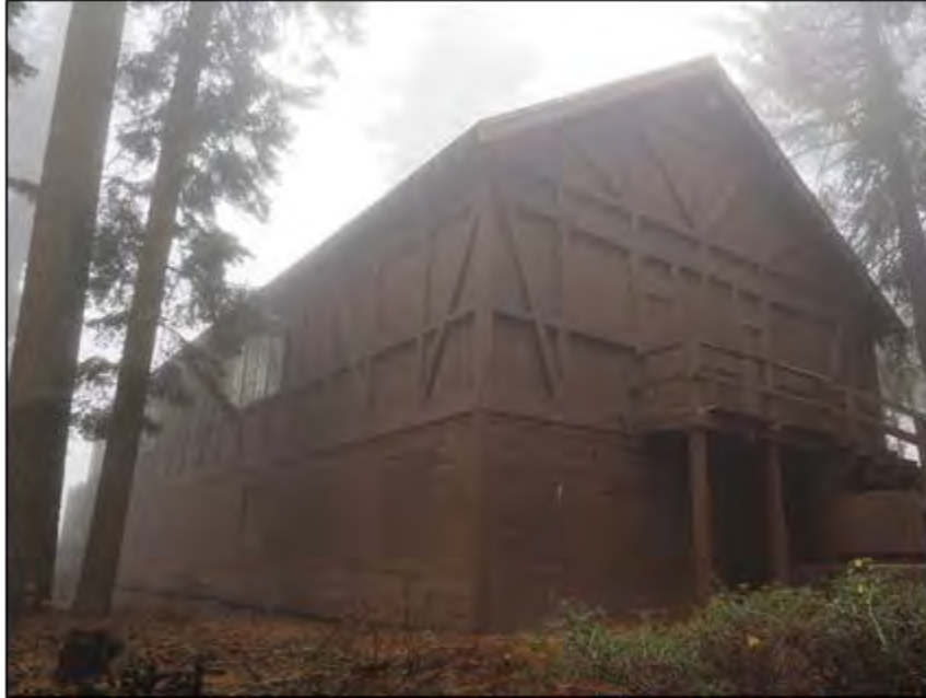
Photo 14 Beetle Rock Building (Assembly Hall). View looking west.
