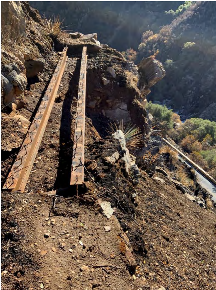
Figure 2. Burned boardwalk, Hospital Rock-Potwisha trail.
