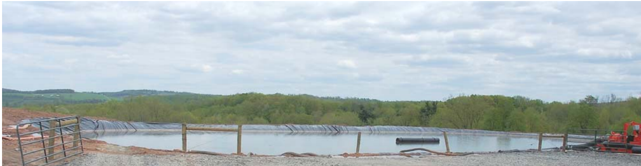
Photo 5.20 c Fresh water supply pond. Black pipe in pond is a float to keep suction away from pond bottom liner. Ponds are completely enclosed by wire fence. Source: NYS DEC 2009.
