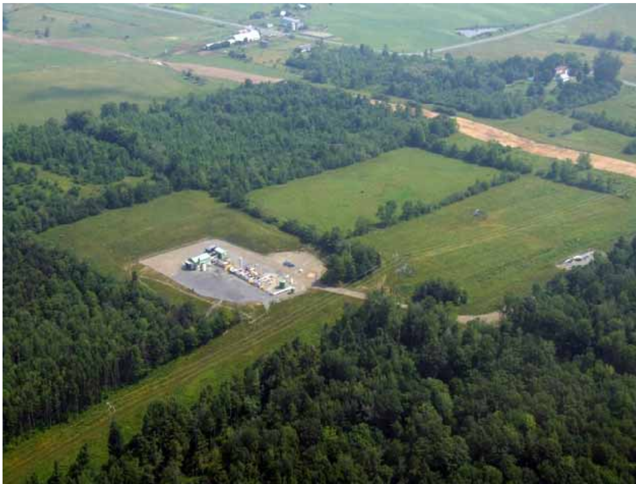
Photo 5.28 - Pipeline Compressor in New York. Source: Fortuna Energy
