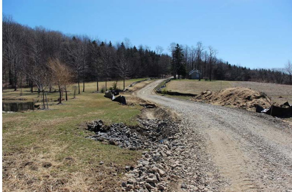
Photo 5.2 Nornew, Smyrna Hillbillies #2H, access road, Smyrna, Madison County NY. Photo taken during drilling phase of improved existing private dirt road (approximately 0.8 miles long). Not visible in photo is an additional 0.6 mile of new access road construction. Operator added ditches, drainage, gravel & silt fence to existing dirt road. The traveled part of the road surface in the picture is 12.5' wide; width including drainage ditches is approximately 27 feet. Portion of the road crossing a protected stream is approximately 20 feet wide. Source: NYS DEC 2008.
