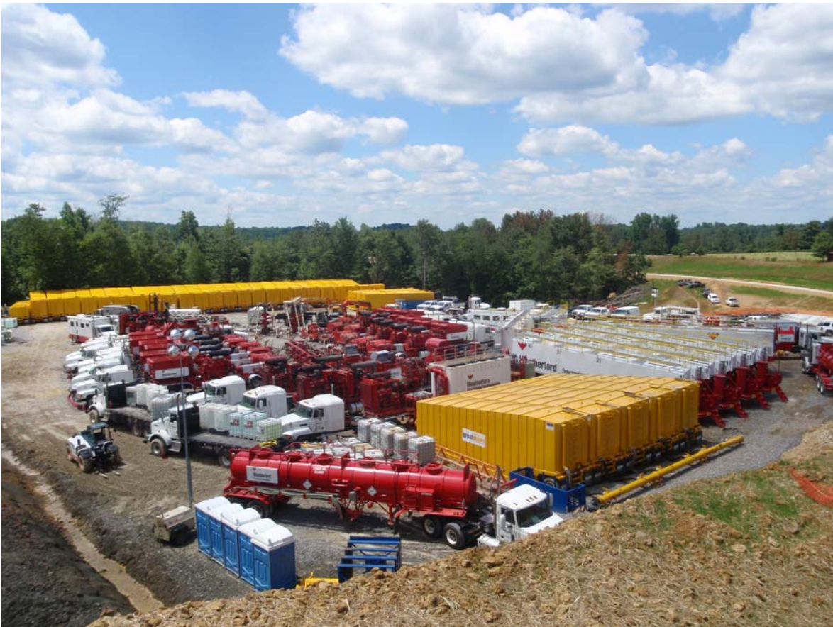
Photo 5.6 Hydraulic fracturing operation, horizontal Marcellus well, Upshur County, WV. Source: Chesapeake Energy, 2008
