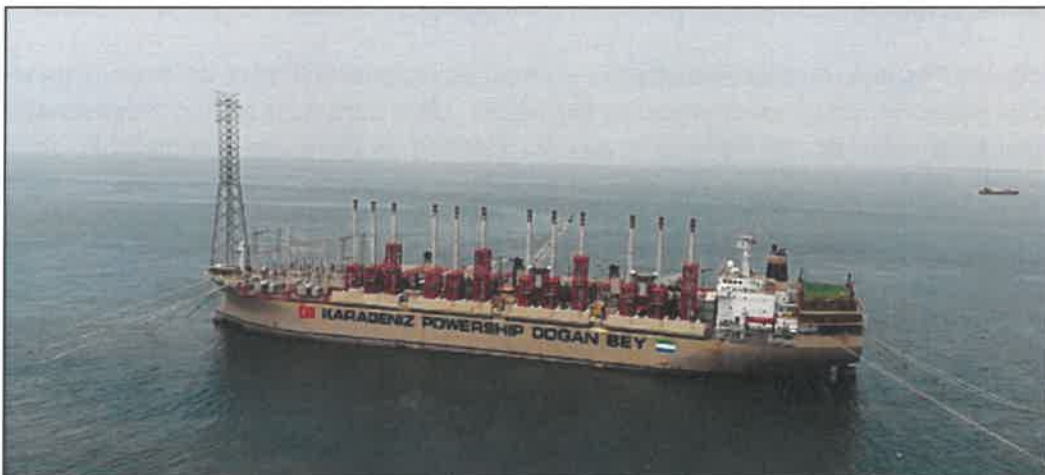
Figure 3-3: Powership mooring system.
