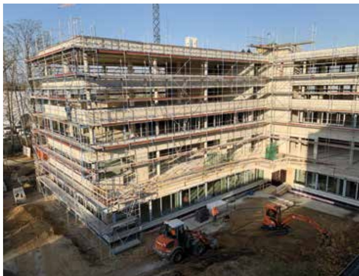
Figure 1 Picture of the CXNS construction site (December 2019).
