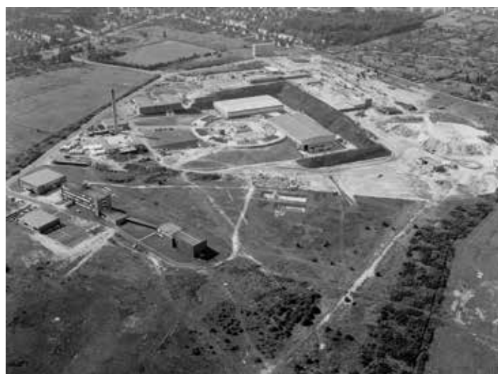
Aerial view of the DESY campus in Hamburg-Bahrenfeld in 1963: The construction of the accelerator ring (centre) is finished, other buildings are still under construction.
