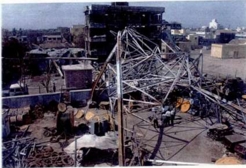
DAMAGED MICROWAVE TOWER PORBANDAR
