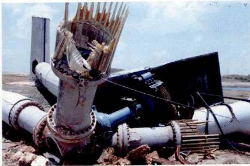
DAMAGED WIND MILLS
