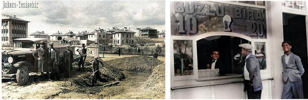
Figure 3.28 Infrastructure works at the intersection of Sakarya Street and Atatürk Boulevard, 1930 (Left). Colorized by the author.
