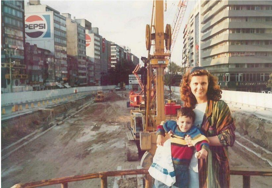
Figure 3.59 Mother and son and ongoing metro construction in Kızılay, 1992.
