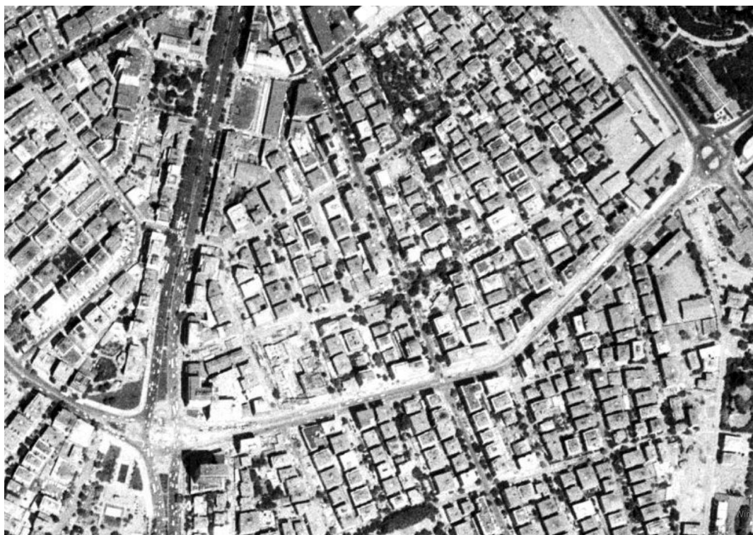
Figure 3.41 Aerial photograph of Sakarya Street and its surroundings, 1978.
