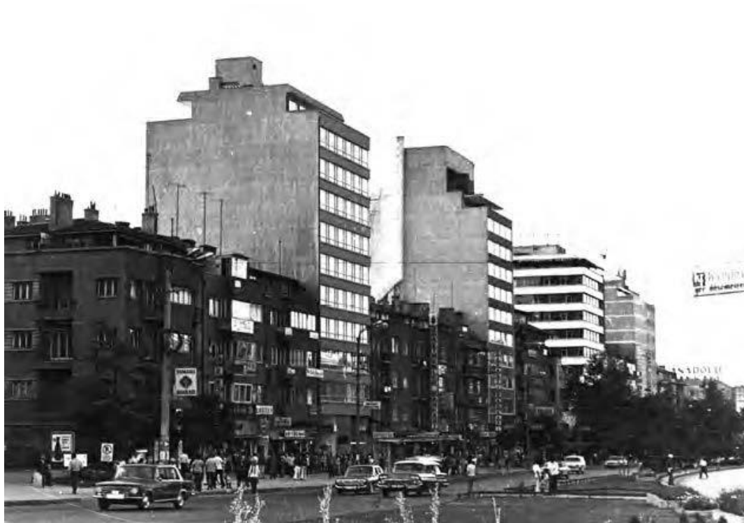
Figure 3.39 Buildings that increase the density on Atatürk Boulevard, 1974.
