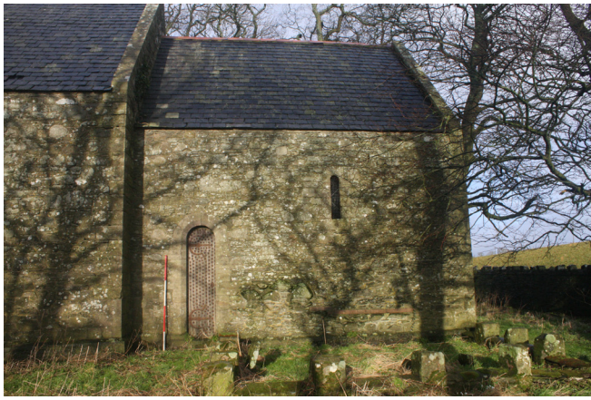
Figure 51: general view to the east side of the south elevation
