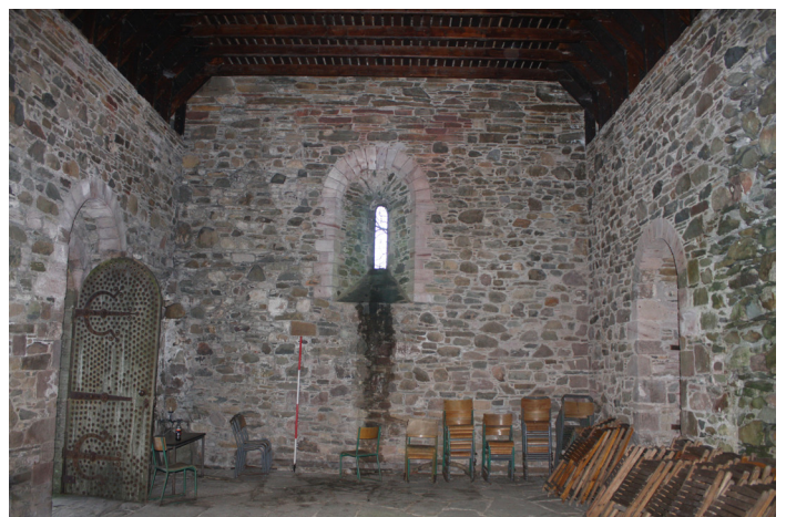
Figure 64: general view of the Nave from the east
