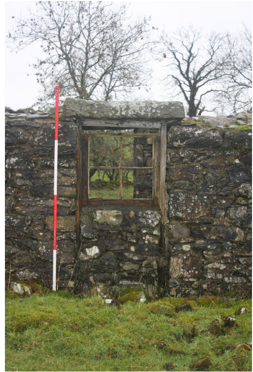
Figure 37: Modified window, Mossend
