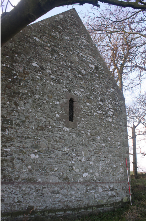
Figure 57: general view of the east gable from the south-east
