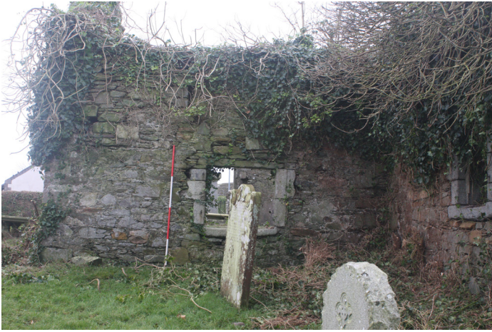
Figure 124: detail of the window to the east of the north elevation, from the north
