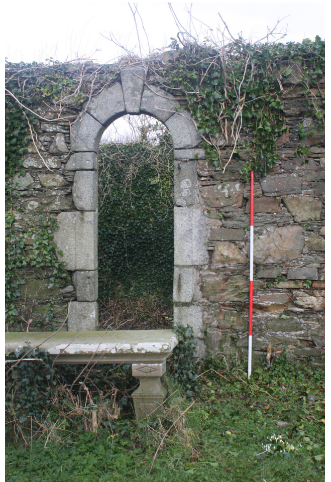
Figure 121: detail of round-headed window on the south elevation, from the south
