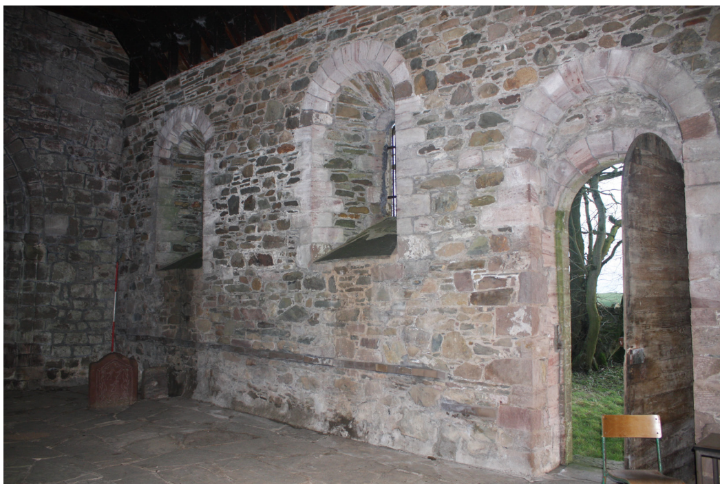
Figure 65: general view of the nave from the north-west
