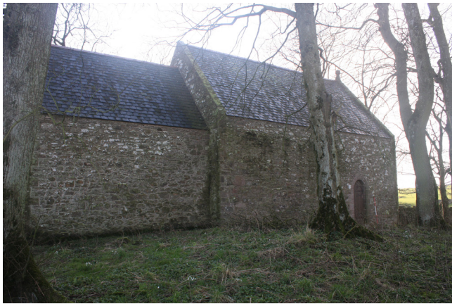
Figure 53: general view from the north-east .
