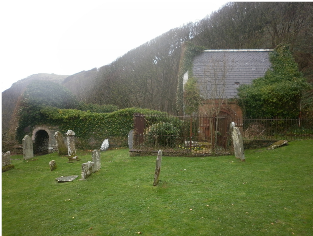
Figure 81: Kirkmaiden Old Church and Graveyard, general view from the SSE
