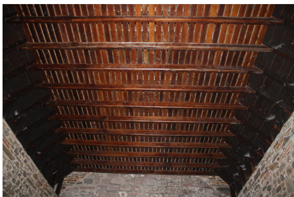
Figure 73: general view of the roof, from the west
