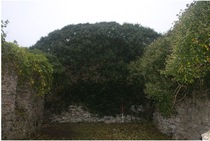
Figure 92: general view of the west wall (interior) from the east
