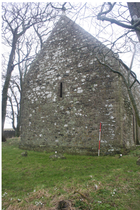
Figure 55: general view of the west gable from the south-west
