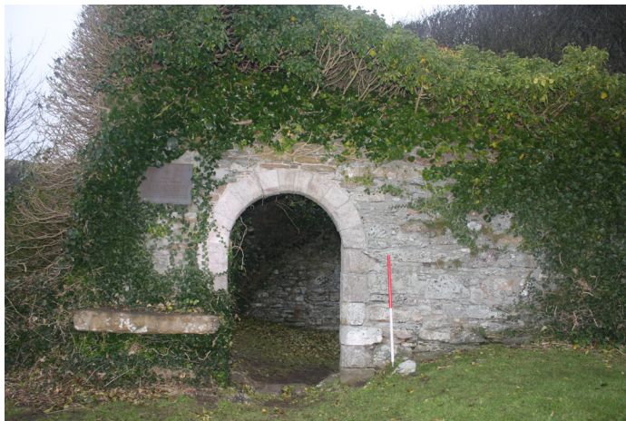
Figure 83: detail of the inserted doorway in the south elevation of the Nave, from the south
