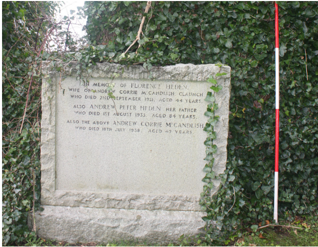
Figure 130: detail of the memorial plaque/gravestone on the west wall of the north transept
