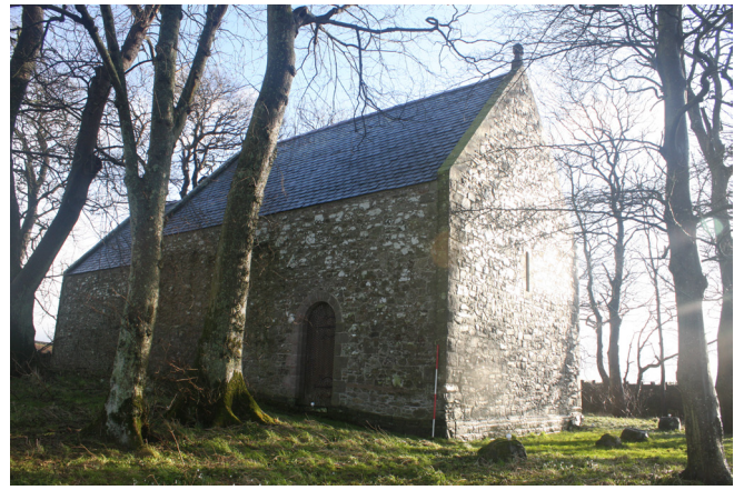
Figure 52: general view from the north-west
