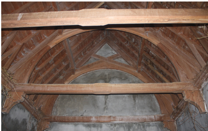
Figure 95: general view of the roof from the west
