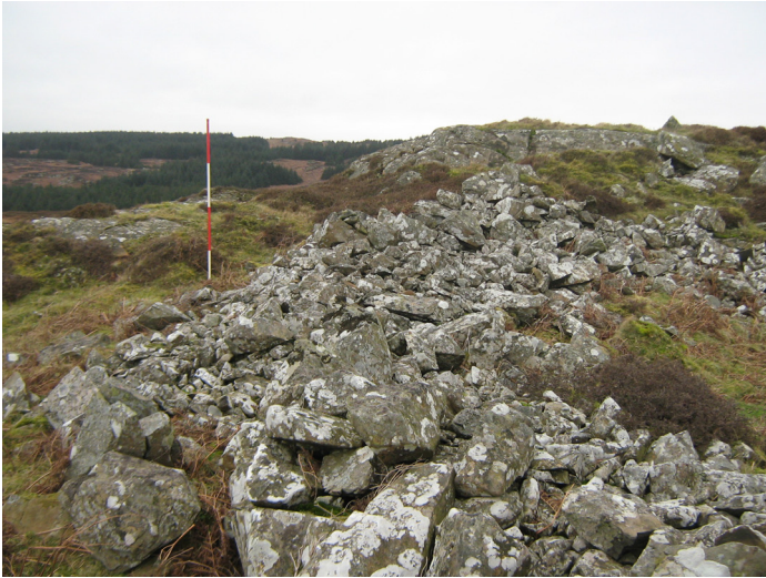
Figure 19: The stone wall of the stone fort at Green House Bridge (MAP 64).
