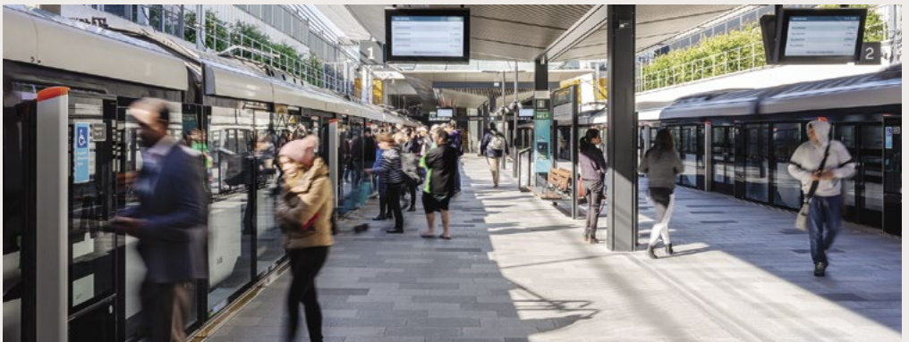
Bella Vista Station, Metro North West Line.
