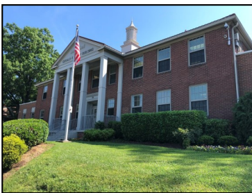
James A. Cayce Administration Service Building
