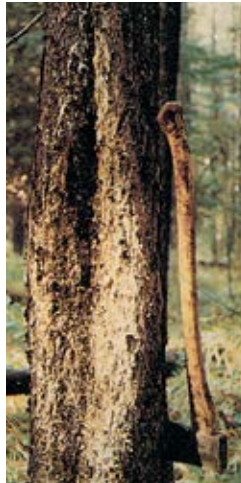
Figure 186. Large sunken cankered area. Main stem is significantly weakened.
