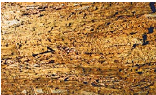
Figure 244. Advanced decay in western larch.
