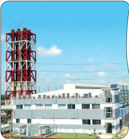
Shikalbaha 105 MW Power Plant
