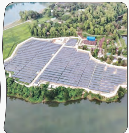
Kaptai 7.4 MW Solar Power Plant
