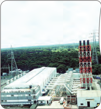
Karnafuli 110 MW Power Plant
