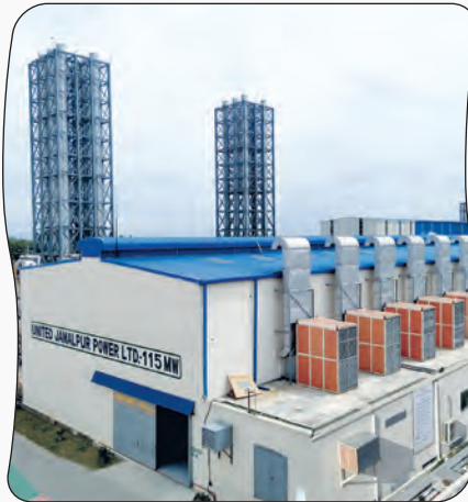
Jamalpur 115 MW Power Plant
