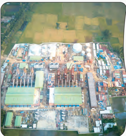
Bogura 113 MW Power Plant
