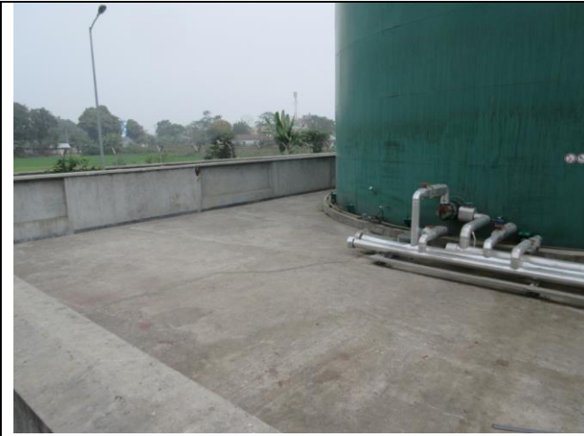
Photograph: Safety bund around fuel storage tanks
