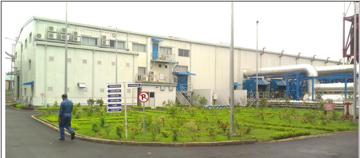
Photograph: External view of the plant (partial)
