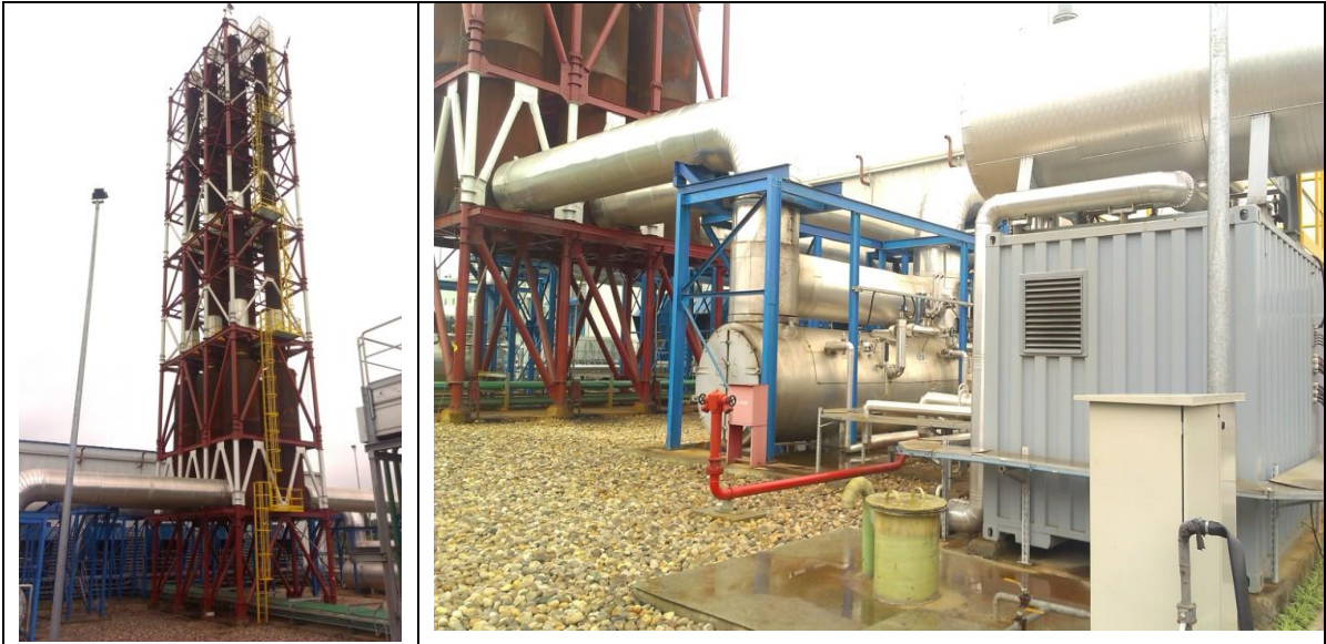
Photograph: Close view of a stack (42 m height) and stack base
