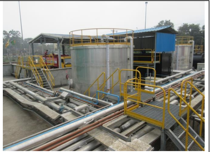
Photograph: Safety bund around fuel storage tanks
