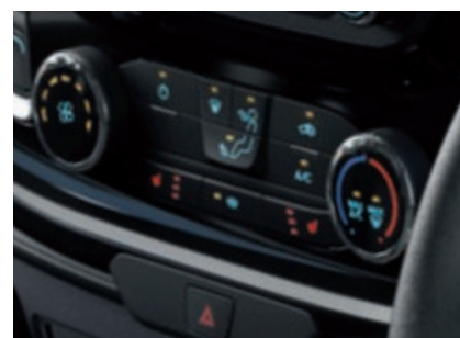
Air conditioning (Standard)
