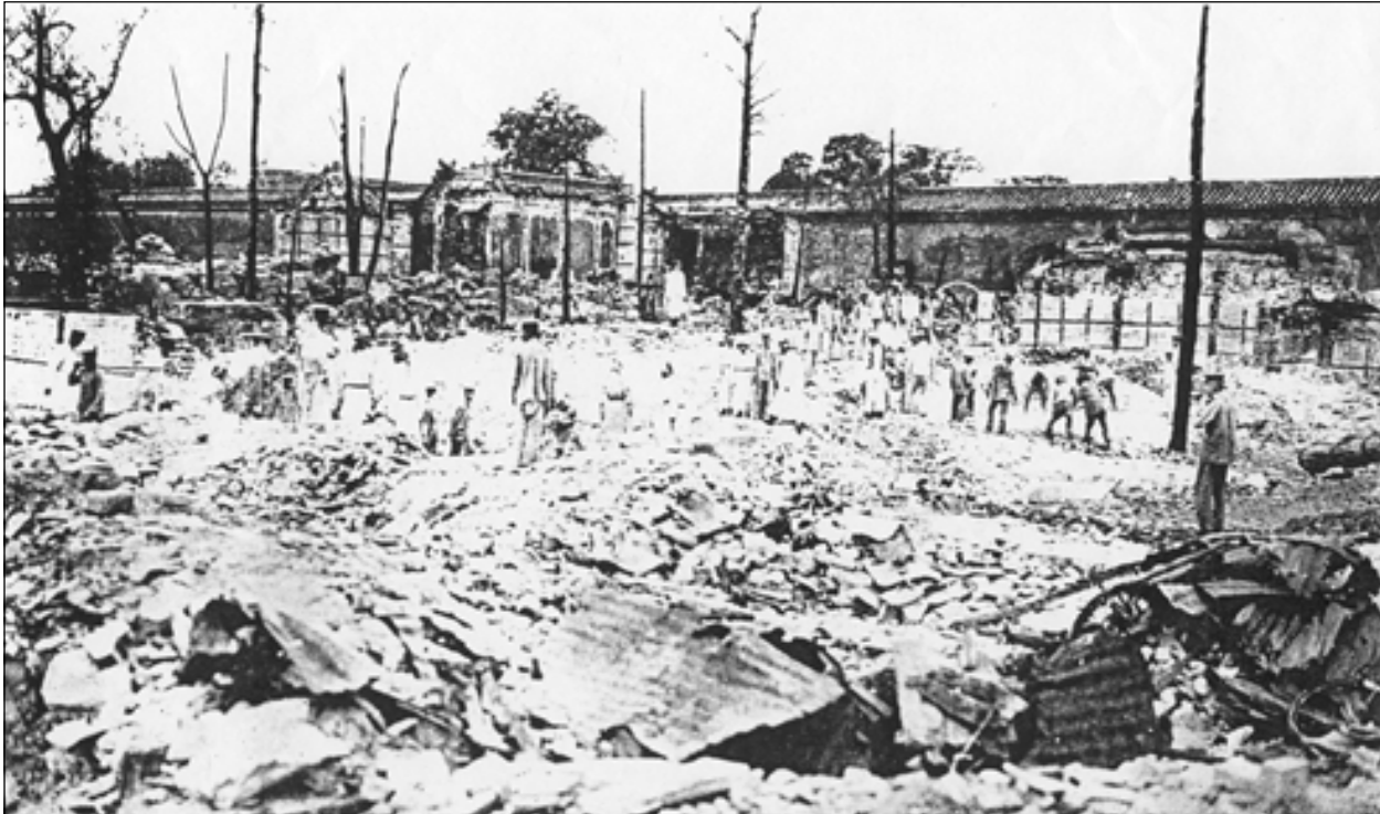
Site of the Palace of Established Happiness after the fire.
