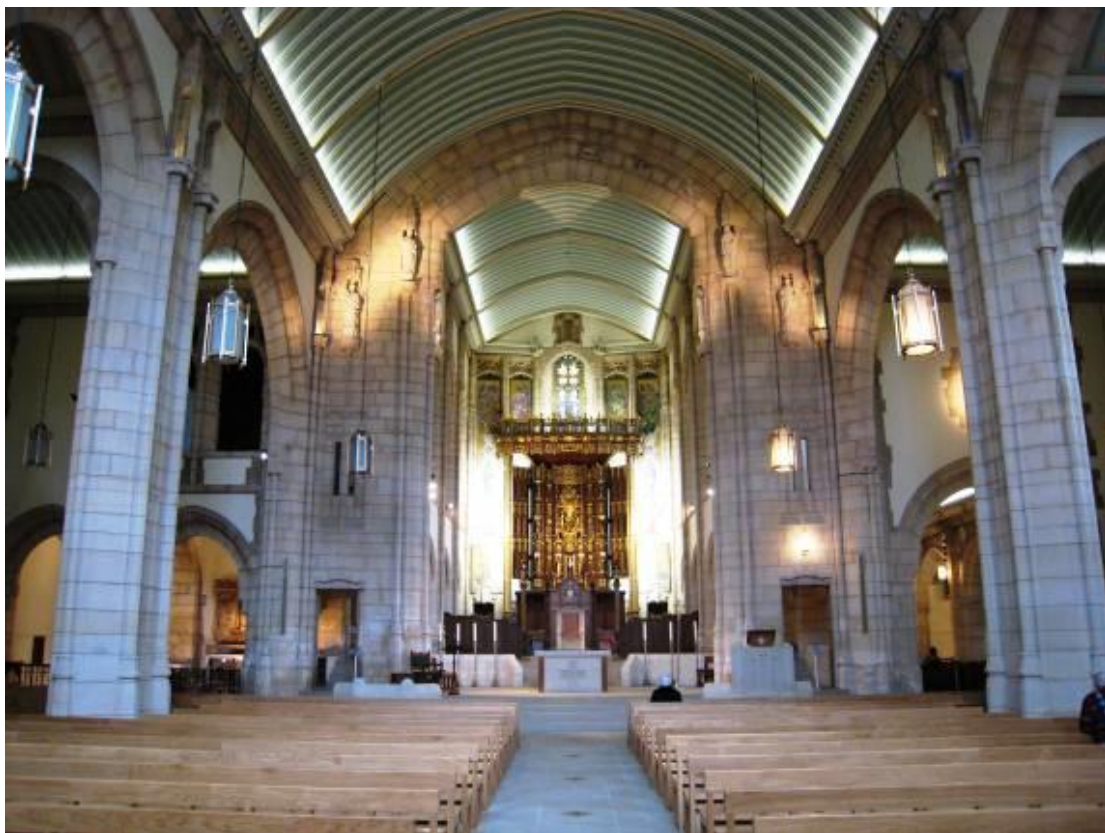
Figure 49: Leeds Cathedral, interior, 2008 (AHP)
