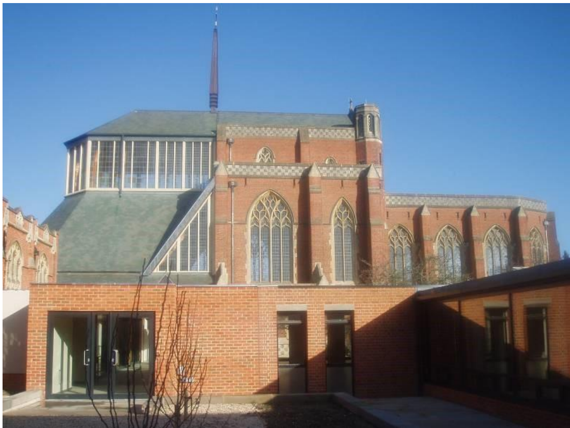
Figure 20: Modern Gothic: Michael Blee's completion (left) of Douai Abbey church, Berkshire, 1992-3 (AHP)
