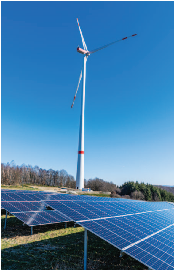
750 kW hybrid PV & Wind system, Gielert, Germany.
