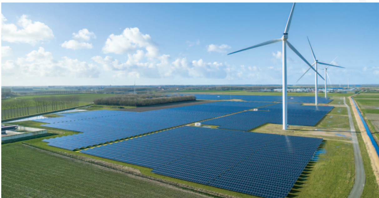
38 MW solar & 22 MW wind, Haringvliet, South Holland, the Netherlands.
