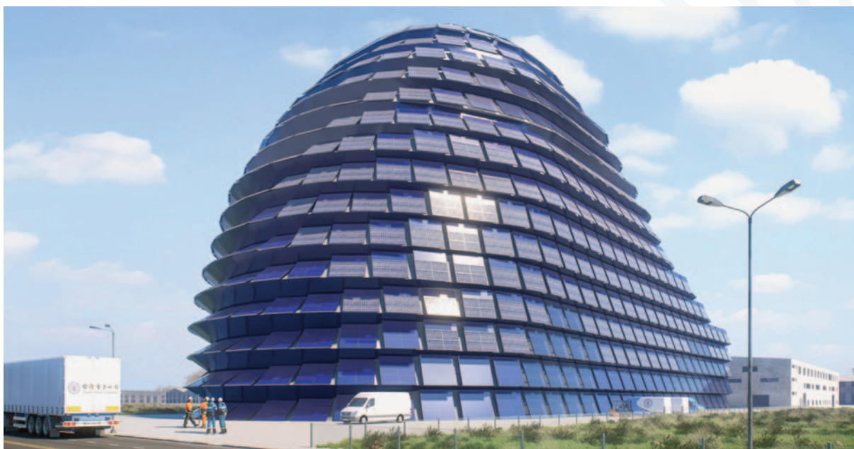
Sun Rock building (under development), Taichung, Taiwan.
