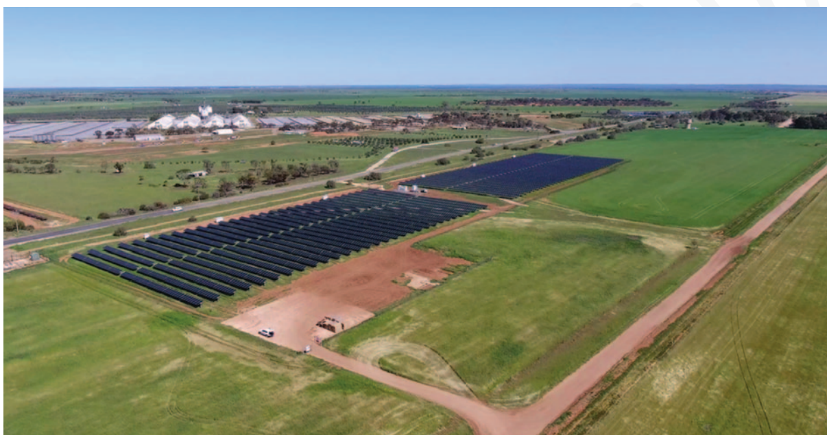
1.9 MW, Bowmen Solar Farm, Australia.
