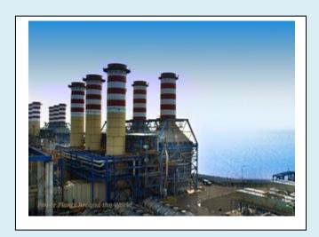
Priok Generation Business Unit is one of generation units owned by PT Indonesia Power. Now, 16 generator units are installed which has 1,248 MW installed capacity consist of two units of opened cycle PLTG (gas turbine power plant); six units of PLTD (diesel power plant); two blocks of PLTGU (combined cycle power plant) which one block consists of three units of gas turbine and a unit of PLTU (steam power plant).
