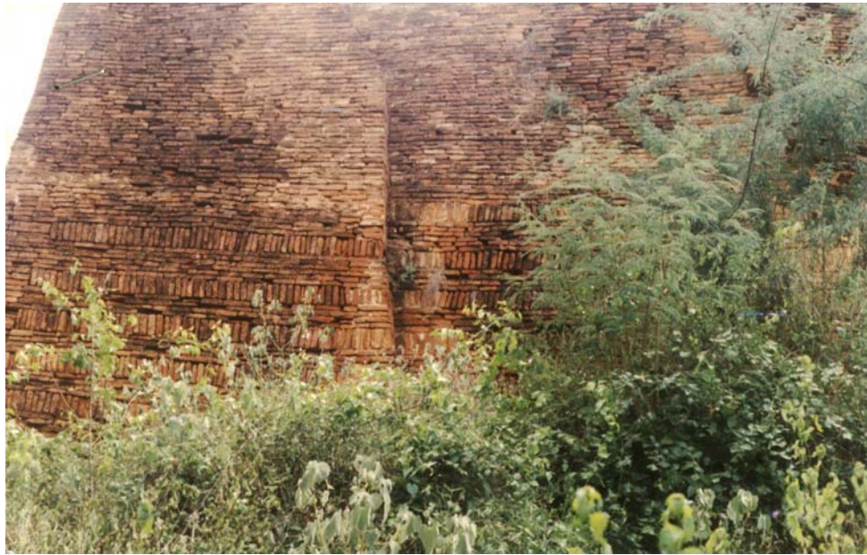
09. Ma Ya Khoe brick bonding pattern, North Wall of Pakhangyi (Photo by Tin Lwin, 20 Sept: 2003)
