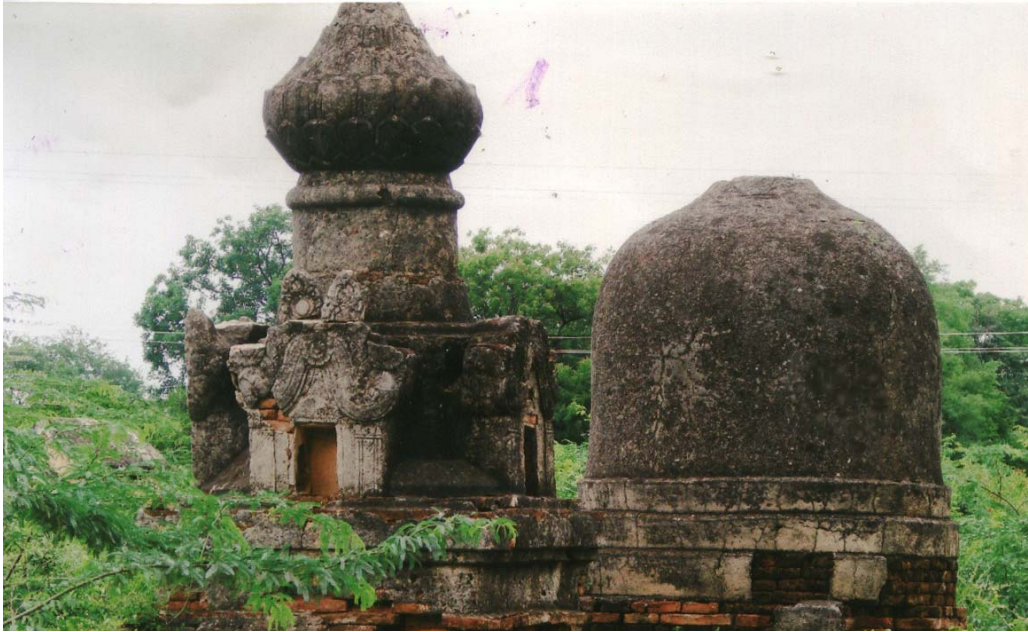
69. Stupa-, Hsin-gu, Kyet-tu-yway Gu, (Elephant and Parrot Caves) (Photo by Tint Lwin, 11 Dec: 2005)
