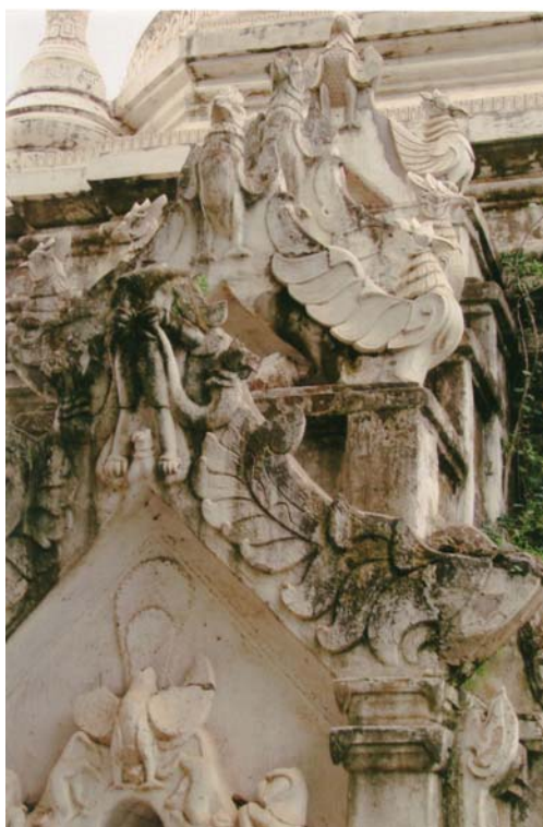
50. Stupa(48), Pyi Lone Chan Thar or Kywet Kywet Hsu, Eastern porch (Photo by Tint Lwin, 12 Dec: 2005)
