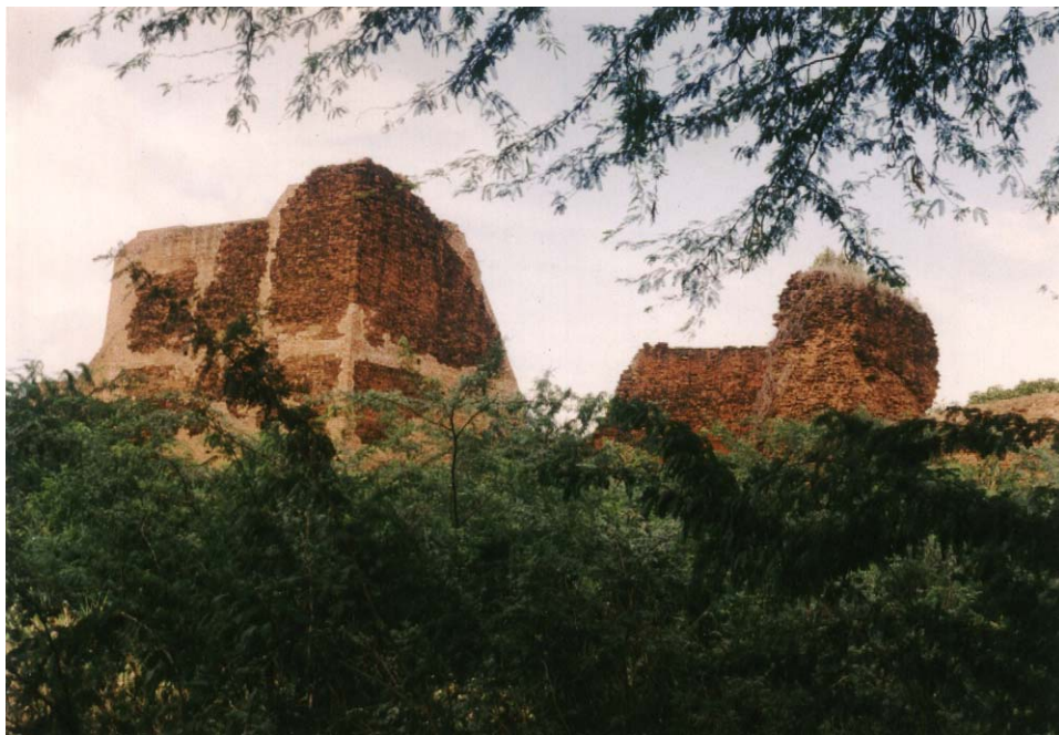
12. West City Wall of Pakhangyi (Khanan Choe Pattern) (Photo by Tint Lwin, 20 Sept: 2003)
