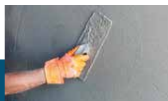
HOUSE Construction & Renovation
