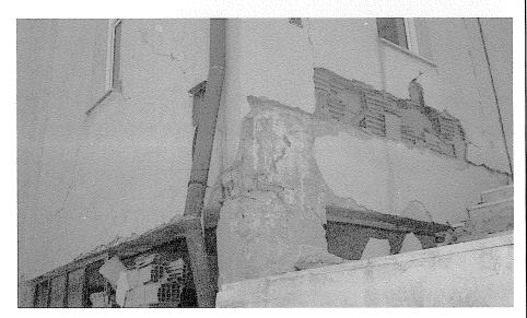
Figure 17 - Damage at a beam-column joint.
