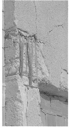
**Figure 12** - Exterior beam-column joint damage.
