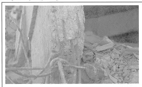
Figure 14 -Bond failure at column base.
