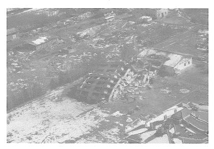
Figure 13 - Collapsed and damaged 8-story apartment buildings.
