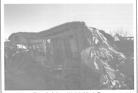
Figure 5 - Collapsed himis building in Eber.
