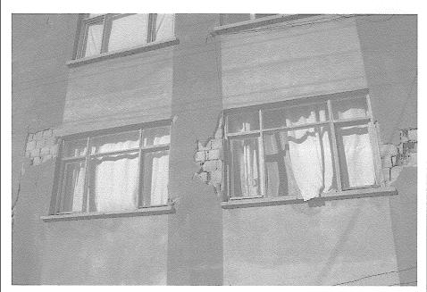
Figure 7 - Heavily damaged 4-story masonry building in Cay.
