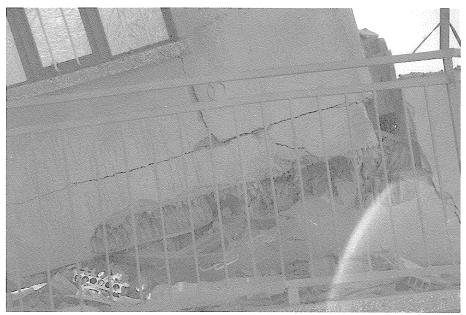
Figure 6 - Collapsed masonry building built with hollow clay tiles.
