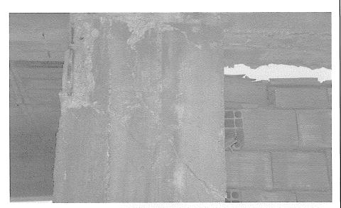
Figure 16 - Observed column shear failure.
