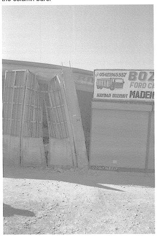
ited beam bar slip, longitudinal column bar buckling, and some level of diagonal tension cracking (Figure 17).
