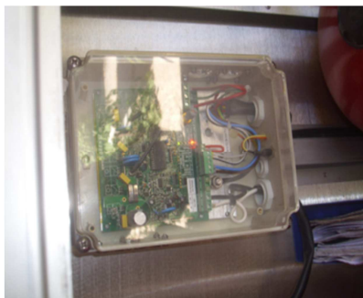
Figure 51: Circuits de commande
