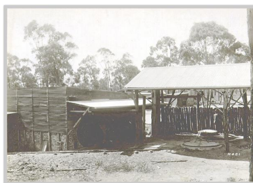
Above: The Wellsford eucalyptus distillery plant. On the right are the vats for steaming the leaves. On the left is the boiler for raising steam. The plant produced about one ton of oil per week.
