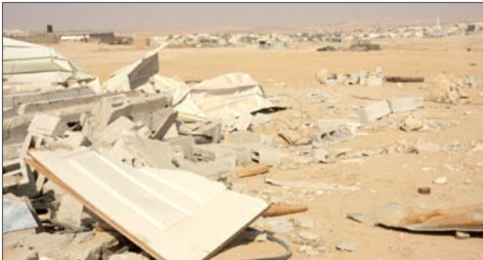
Demolished structure that was home to a family of 8 Palestinians. Segev Shalom concentration township in the background (Anne Paq, ©Badi).
