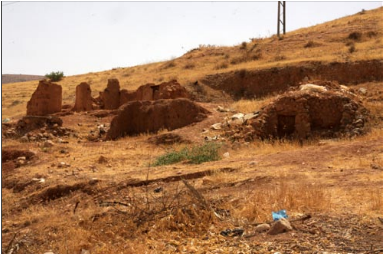
Palestinian Home in Furush Beit Dajan (Area C). The home was built before 1967, and therefore 'legal' - but when it collapsed, Israeli authorities banned the owners from fixing or renovating the home, forcing the family to live in a tent nearby. (Anne Paq © Badi)
