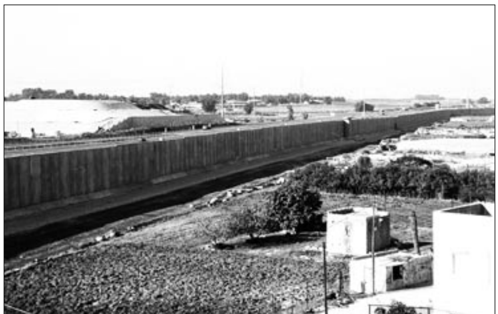
The Wall on the western side of Qalqilya. On the other side of the wall, the Trans-Israel highway (© Anne Paq)
