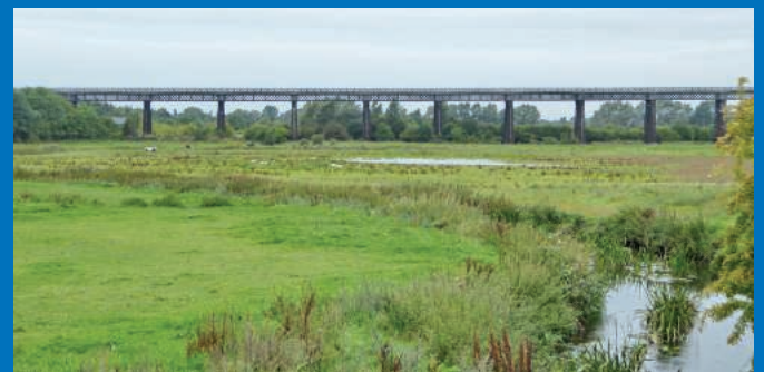
Bennerley Viaduct – centre-stage for preservation at the festival this year.
