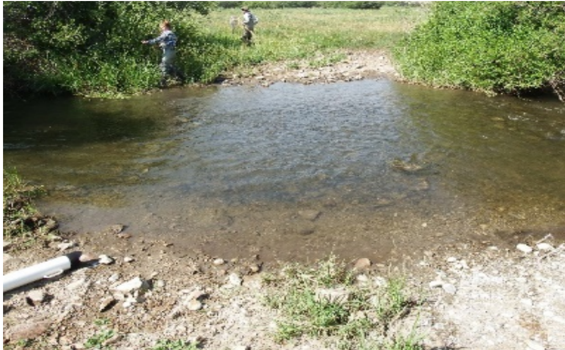
Figure 6-6. Unpaved crossing at site MDLG06-05a
