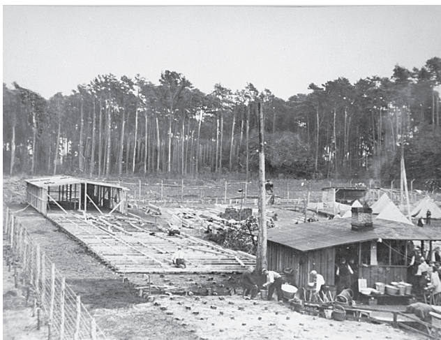
Prisoners erect the barracks foundations at Stutthof, September to October 1939, at which time the camp was not part of the Inspectorate of Concentration Camps (IKL).
