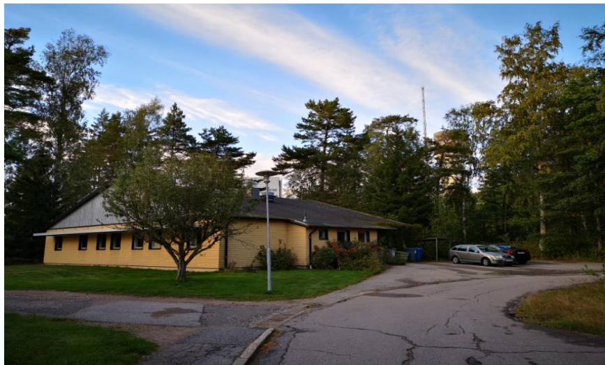
CNNC Nordic R&D Center on-site office at Studsvik Technology Park
