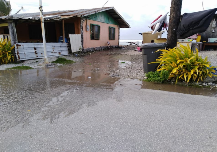
Picture. 2: Tides and Inundation pictures in Majuro during February 3-4 high tides (top: inundated roads, bottom: inundated houses). Event is associated with northerly swell from northern Pacific storm. (Photo Credit: Mr. Charles C Guard).
