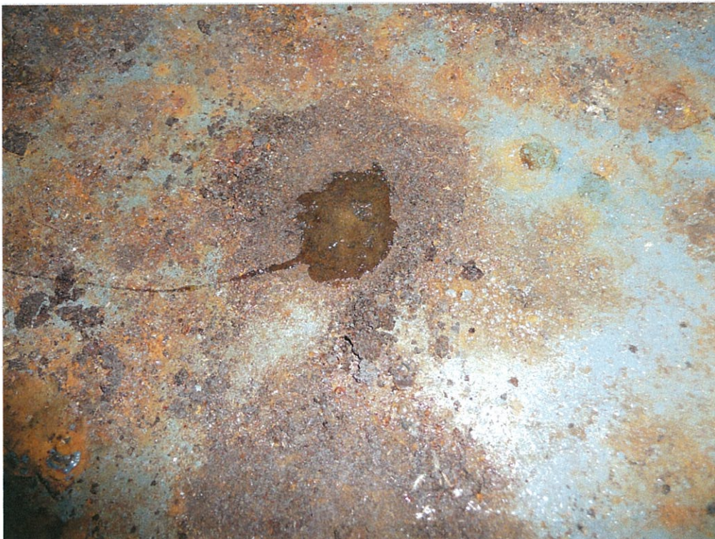
Figure 3: Area of corrosion on the headstock floor on EMU 23
