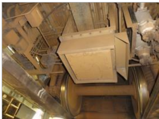
Figure 76 Image of ATP antenna
