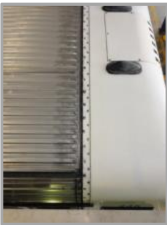
Figure 90: Image of roof panels
