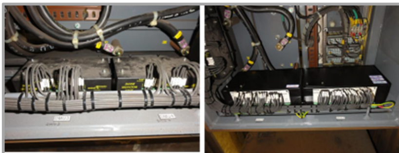
Figure 72: Image of door control unit
