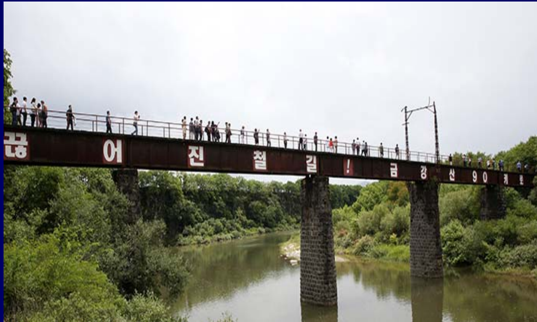
Tourists walk along the Geumgangsang Mountain Electric Railroad Bridge
