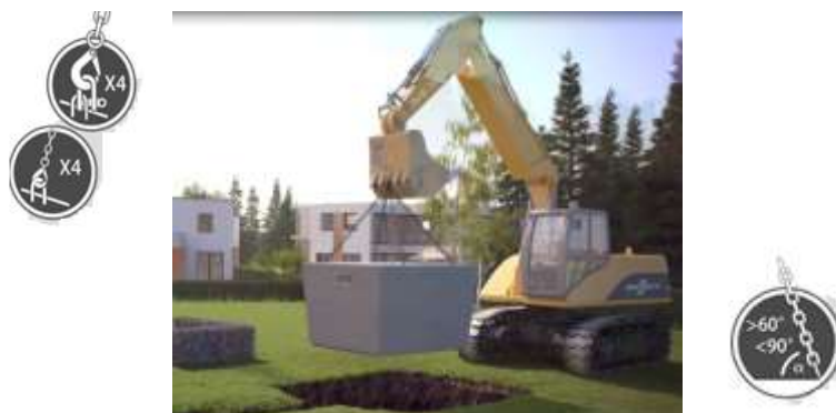
Fig-15: Handling of the tank
