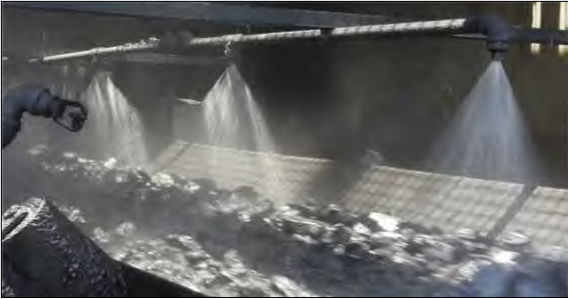
Figure 4.3 : Dust Suppression System at Raw Material Handling Area
