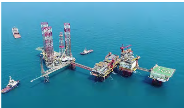
OMV Petrom and Romgaz are developing the Neptun Deep natural gas deposit in the Black Sea. / OMV Petrom
