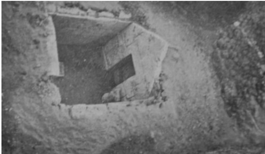
Figure 72: Triangular-pitched roof of Tumulus B at Karalar (Image source: Arık, “Karalar Hafriyatı,” Fig. 25)
