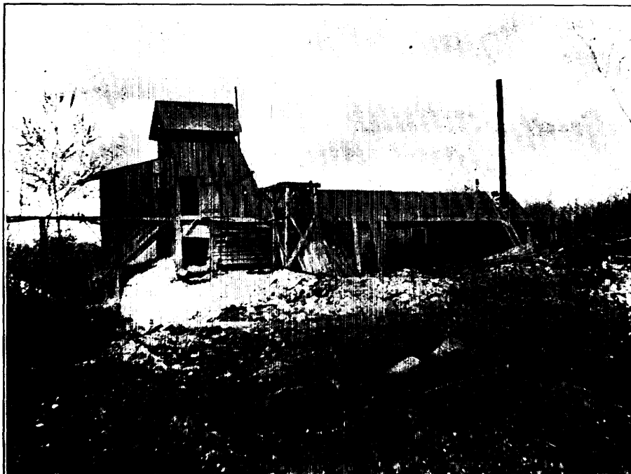
Shaft house, Star of the East gold mine.
