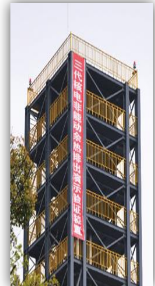
Passive residual heat removal test for secondary side
