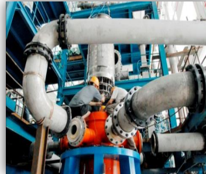
Flow-induced Vibration Simulation Test of Reactor Internals
