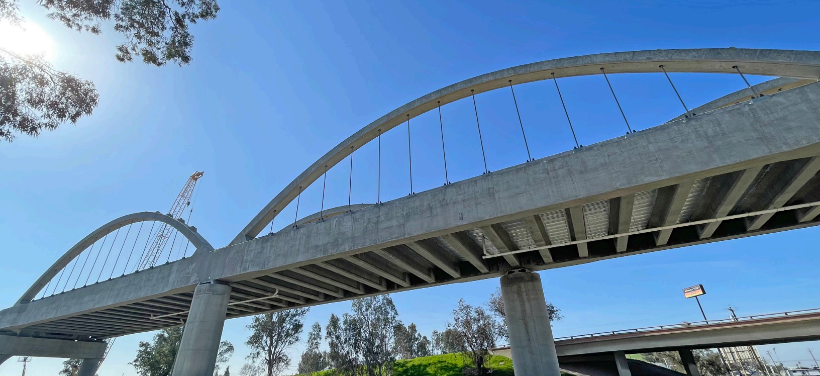
Photo: Cedar Viaduct
