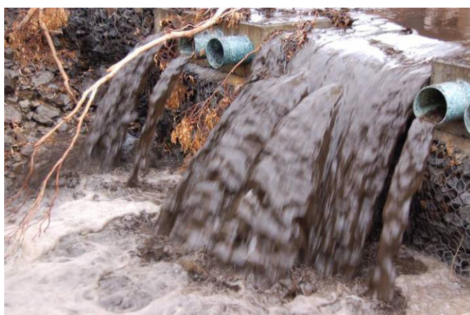
Plate 6. Sediment mobilisation in Leary's Creek (downstream of Robertson's Gully), and damaged Trout barrier, Marysville township, April 2009
