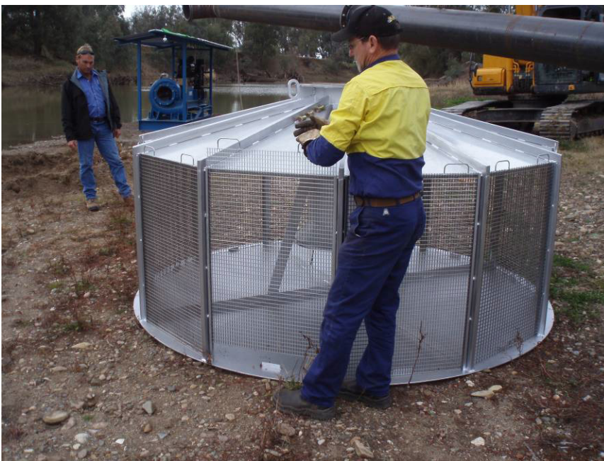
Figure 1: Final screen design showing removable mesh panels that will allow both the aperture size to be changed and the surface area of screen to be adjusted.
