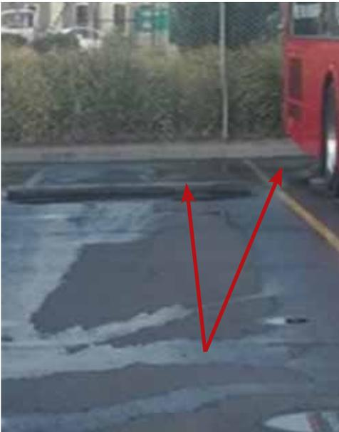
Concrete speed bumps or chocks installed to prevent the bus rolling away.
