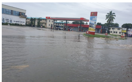
Figure 16: Nadi town inundated with floodwaters on 17 th February, 2023. Source: fijivillage
