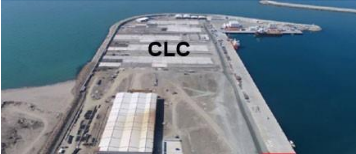
Figure 3: Aerial View of the CLC
