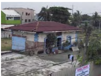
Old Station Building
