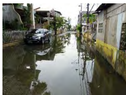
Road Flooding at West Side of Highway
