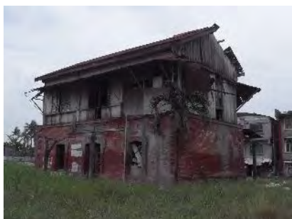
Old Station Building
