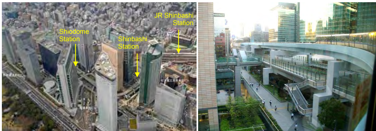
Entire Area of Shiodome Shiosite (Redevelopment Area)
