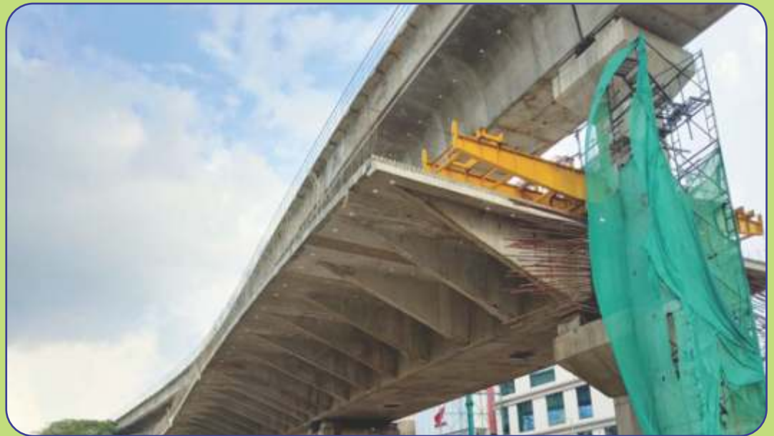
Road segment erection in progress - Reach 5
