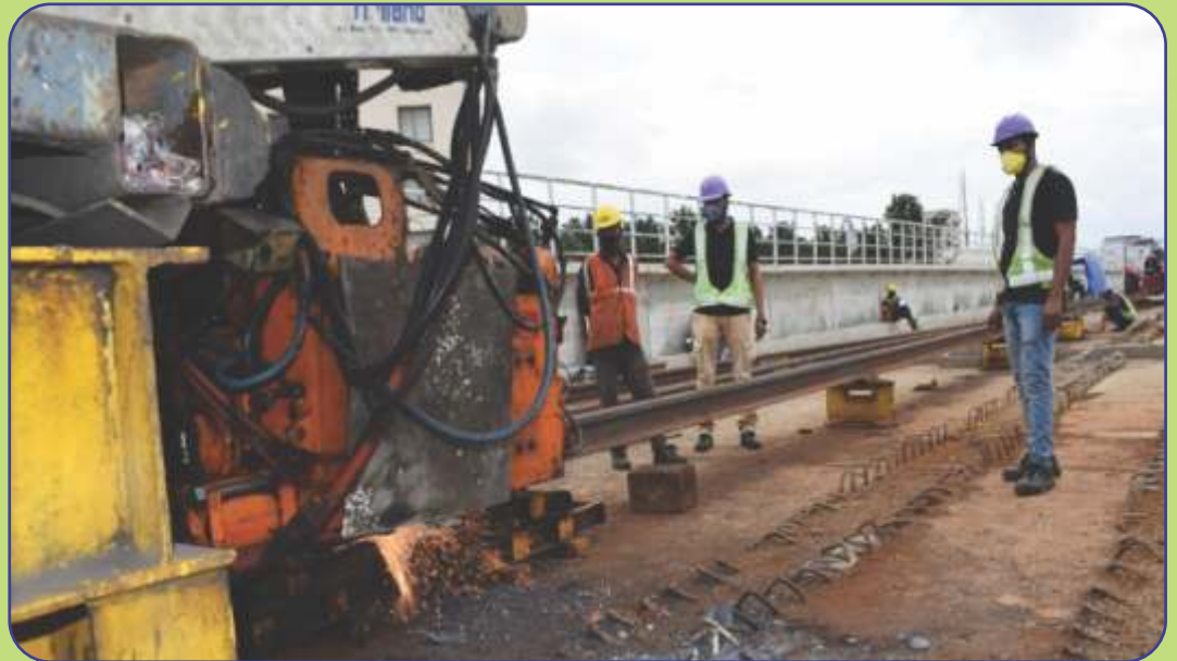
Flash Butt welding work at Reach - 1 Extension
