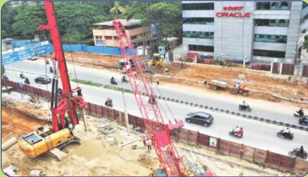
Piling work in progress at launching Shaft Area - Reach 6
