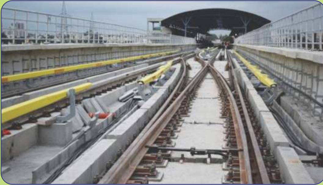
Completed track work along Viaduct of Reach - 4B
