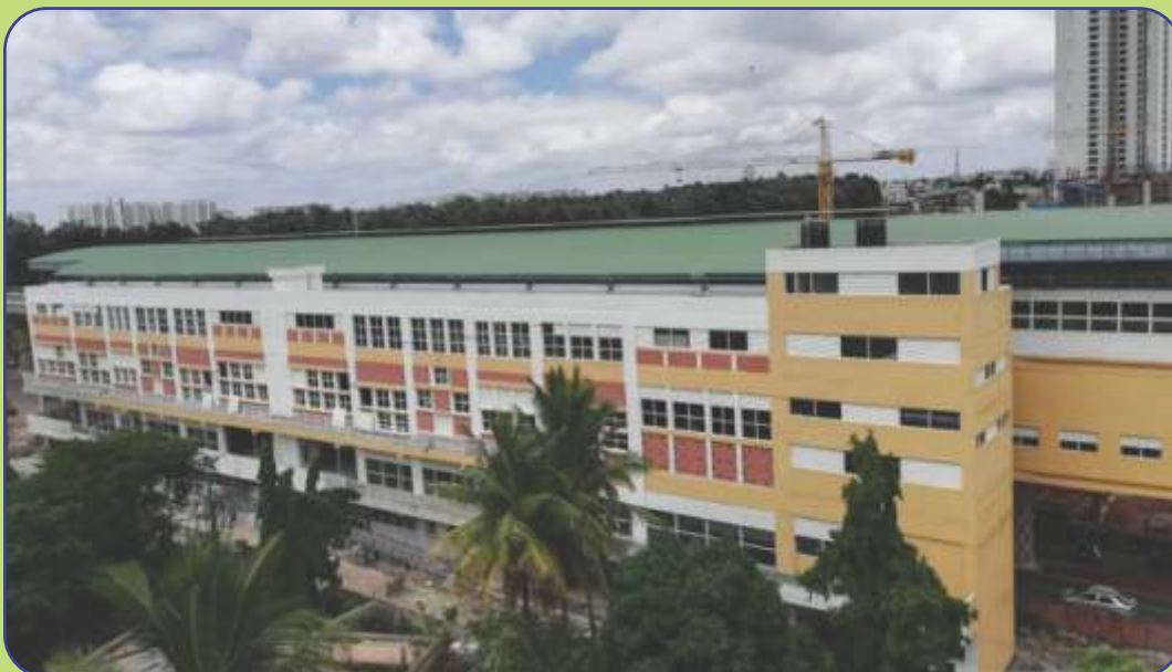
View of Konanakunte Cross Station of Reach - 4B
