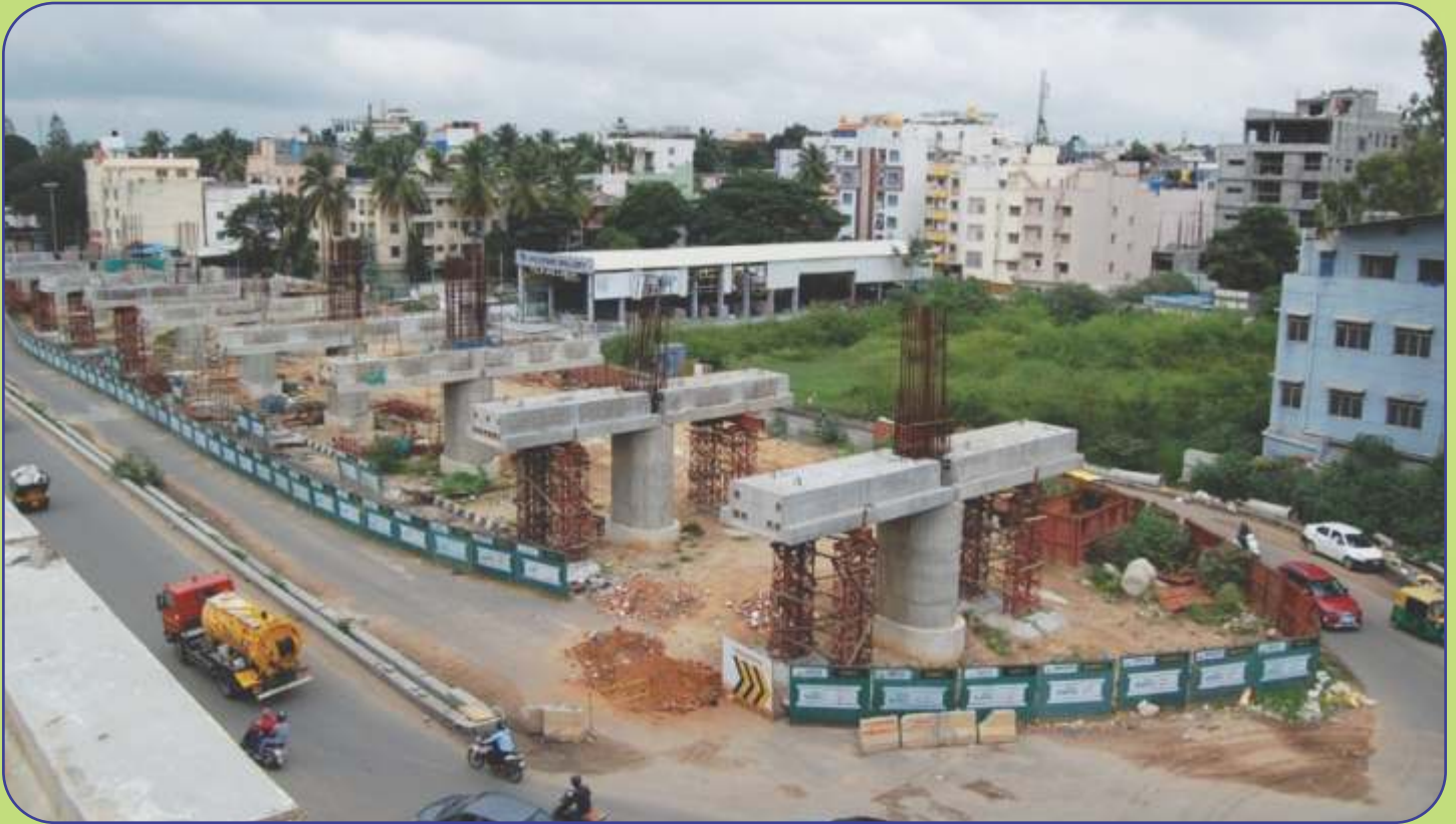
Under Construction of Tavarekere Station
