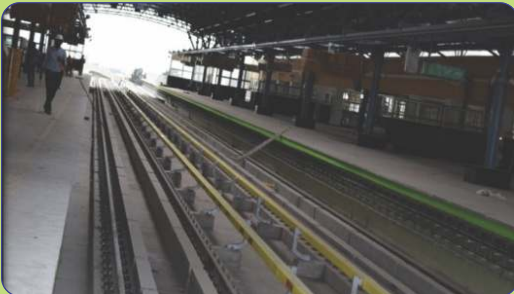
Completed track work along Reach - 4B
