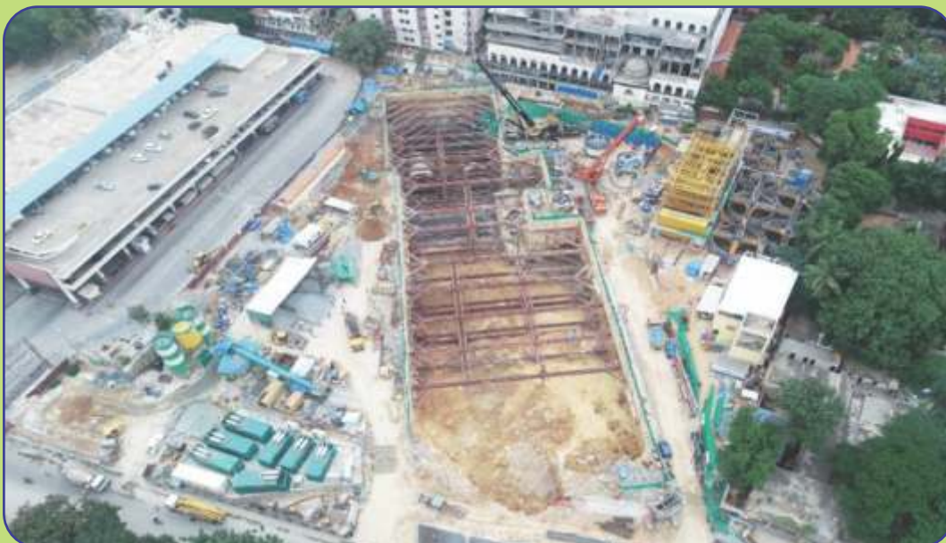
Aerial view of Shivajinagar Underground Station - Reach 6
