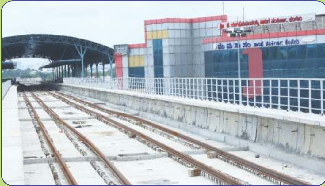
Track laying work in progress in Reach - 2 Extension
