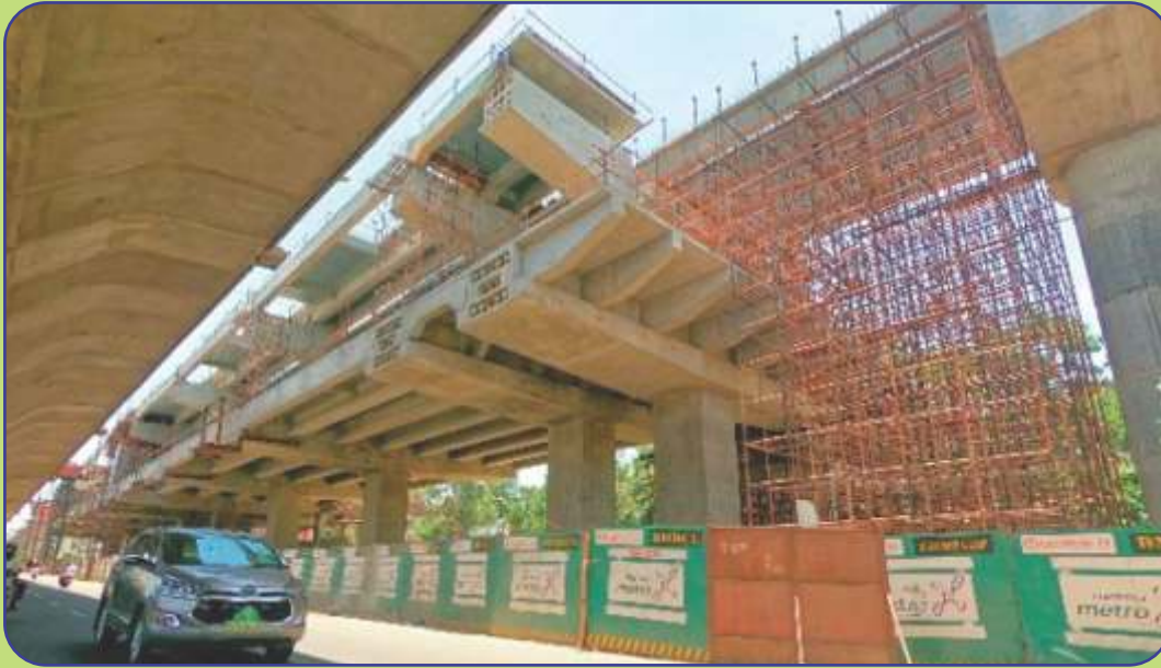
Station work in progress at Reach 5
