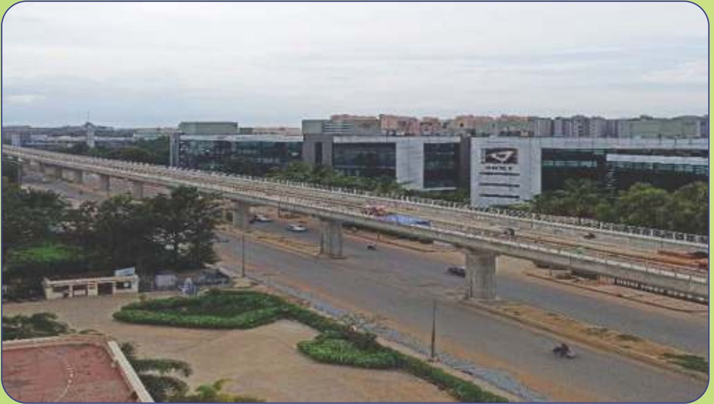
Viaduct completed along Reach - 1 Extension
