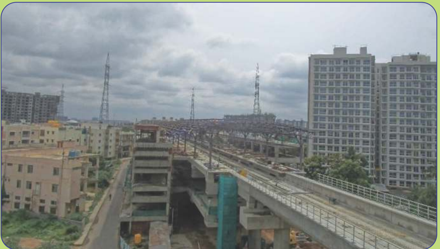
Reach - 1 Extension : Hoody Junction Metro Station works
