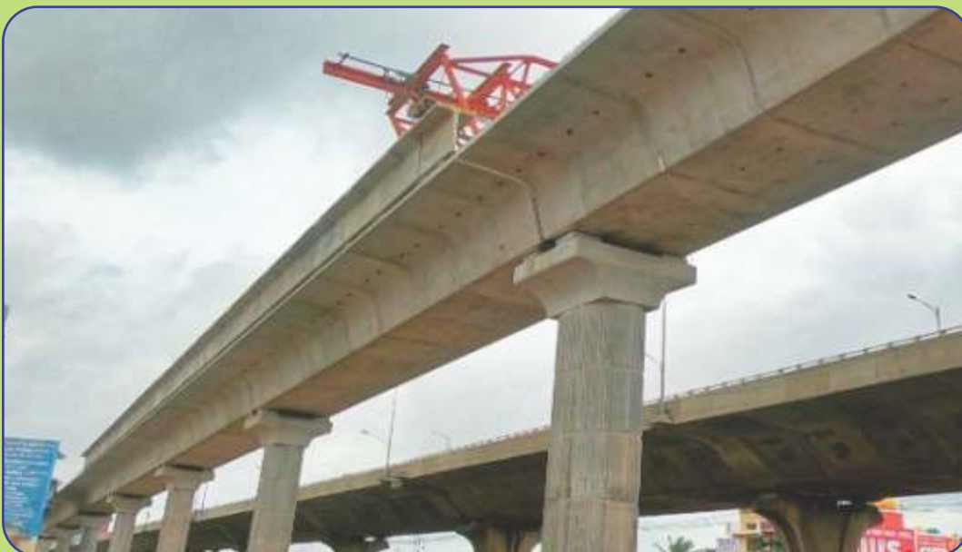
Progress of Viaduct Works in Reach 5
