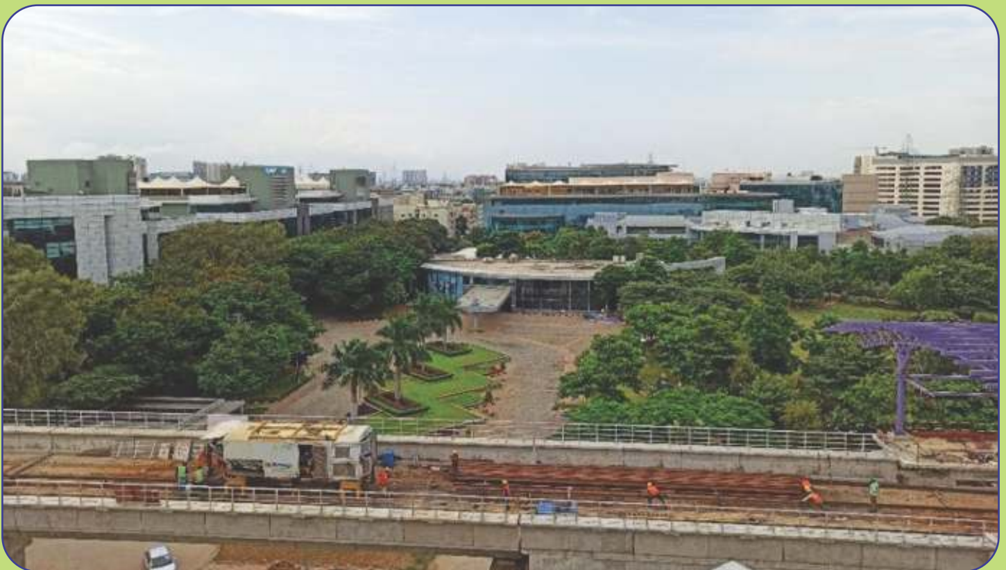
Track work view along the viaduct of Reach - 1 Extension
