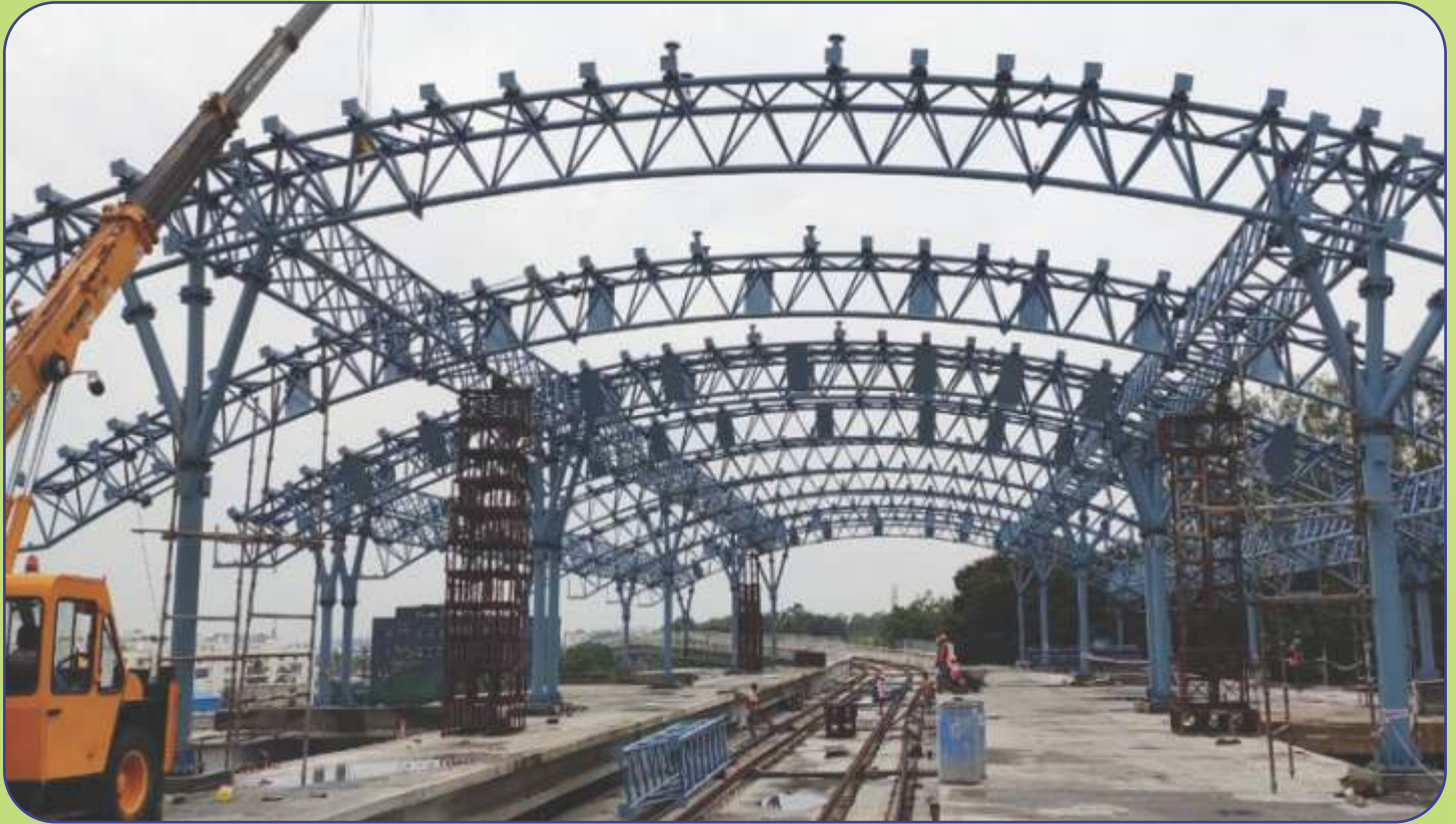
Structural Steel work in Rajarajeshwari Nagar Station in Reach - 2 Extension
