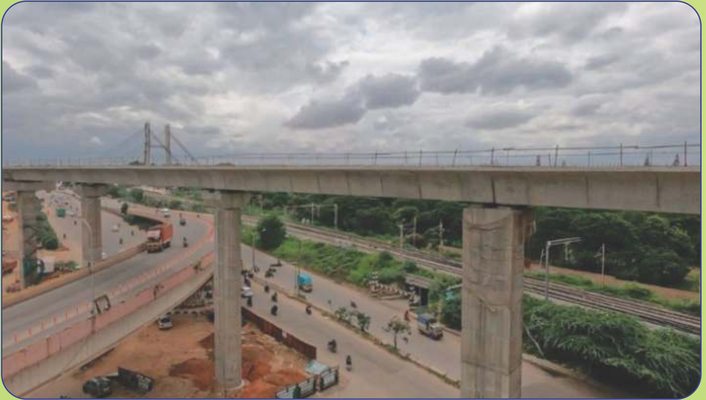
Reach - 1 Extension Metro Rail over ORR Flyover at K. R. Puram Junction
