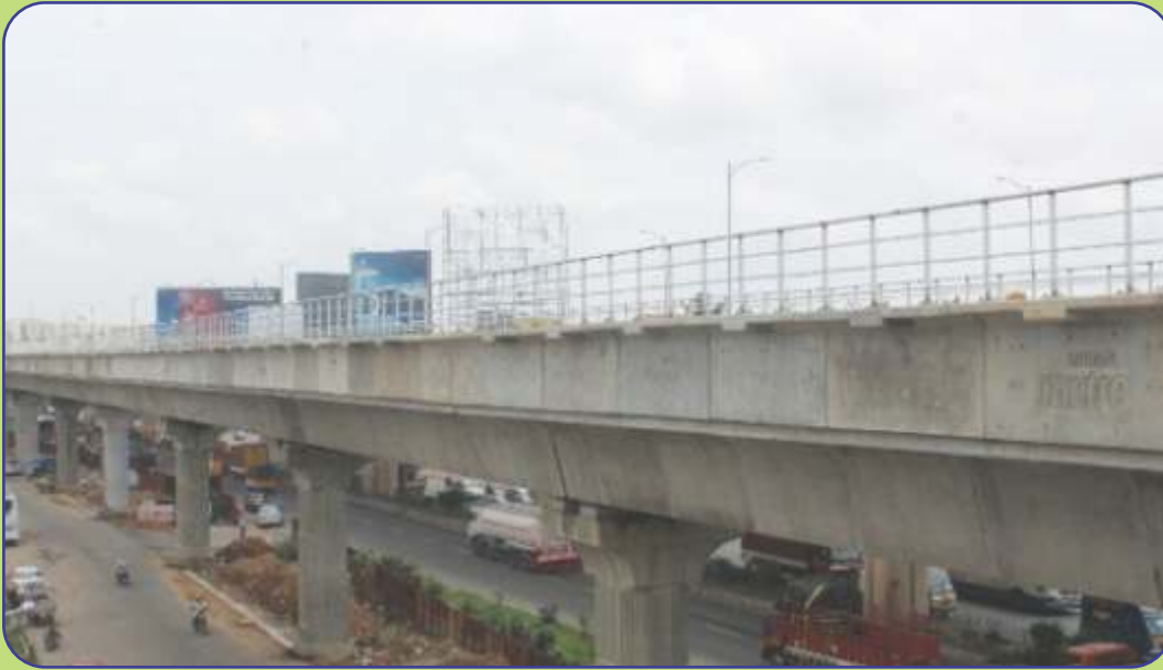
Erection of Parapet Wall and Hand Rail work in progress - Reach 5
