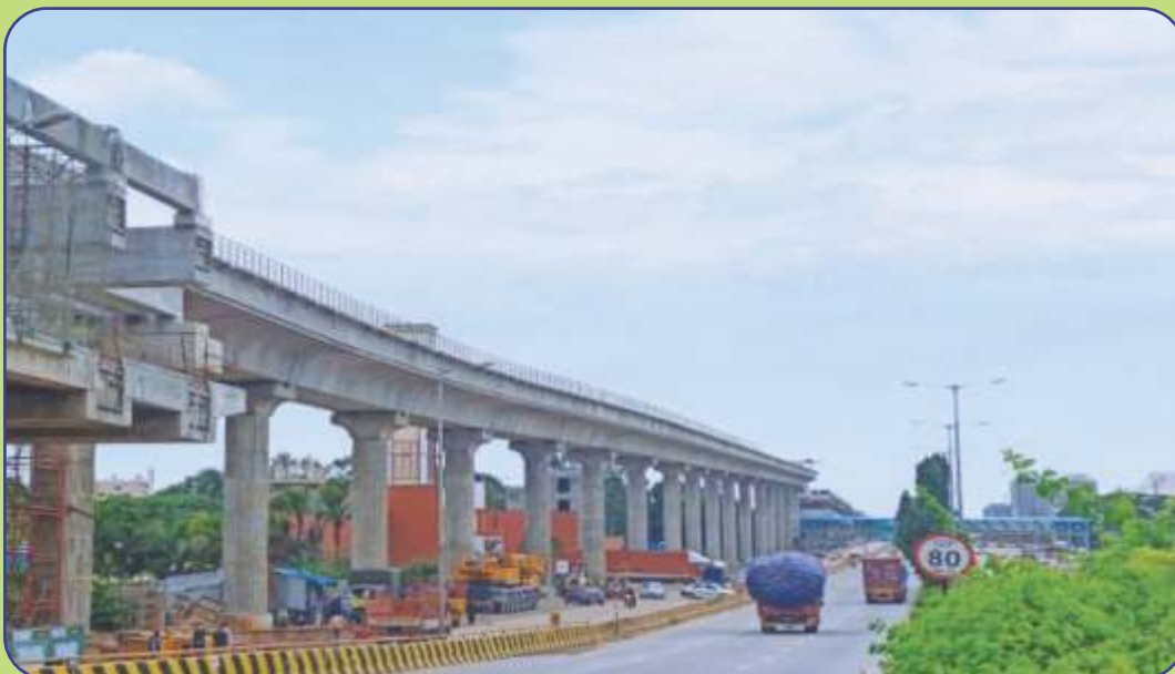
View of viaduct work in progress in Reach - 3C
