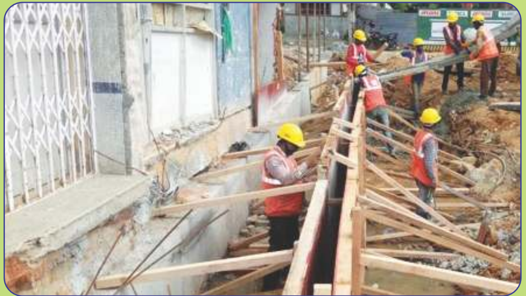
Storm water drain concrete work in progress at Dairy Circle Reach 6
