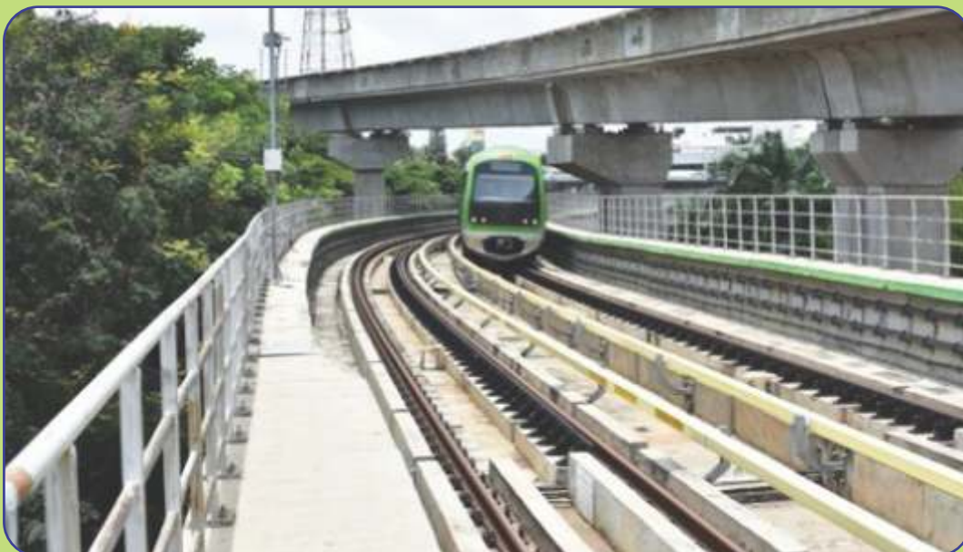
Reach 5 Metro Line cross over in Reach 4 Metro Line at RV Road Station
