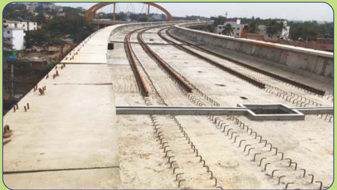
View of viaduct track laying work in progress in Reach - 2 Extension
