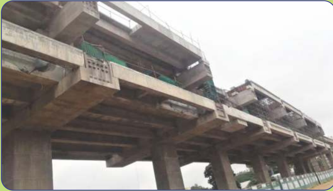
Work in Manjunath Nagar Station Ground Level View - Reach - 3C
