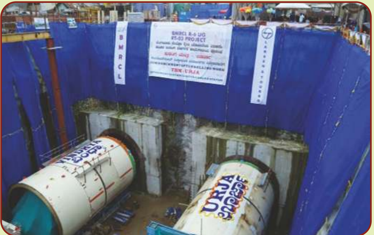
Tunnel Boring Machines 1 & 2 Assembly in progress in Cantonment Station.
