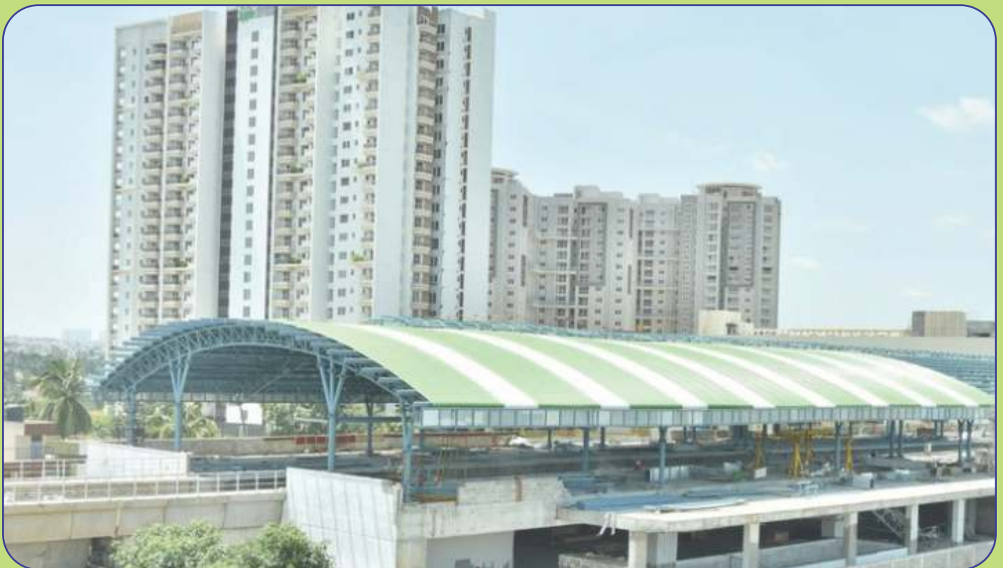
Side view of Nayandahalli Station in Reach - 2 Extension
