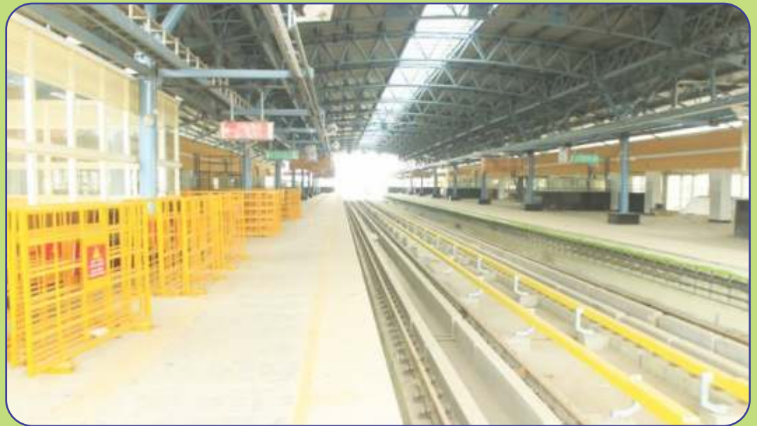
Platform Level View - Anjanapura Station
