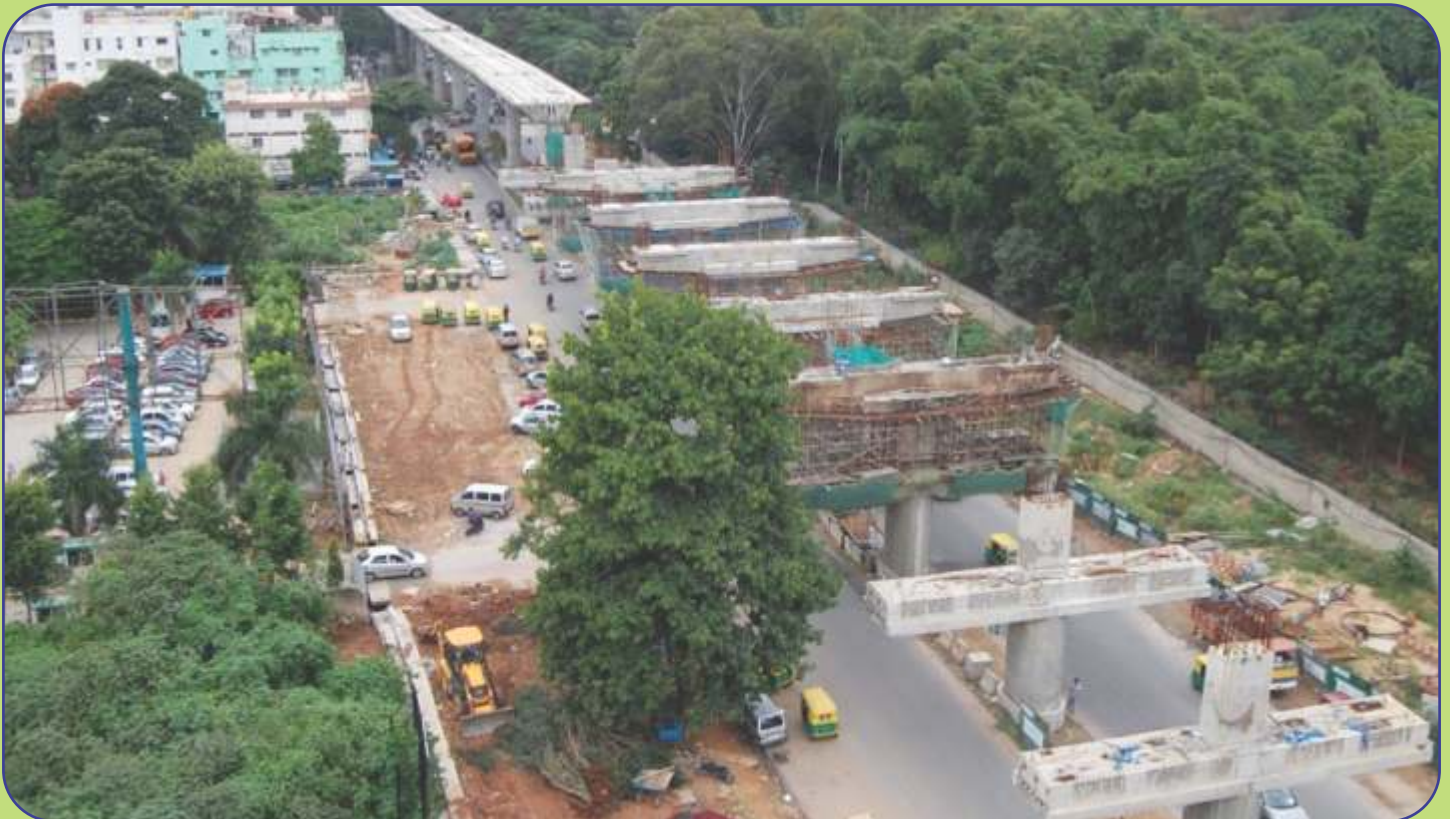
Under Construction of IIMB Station
