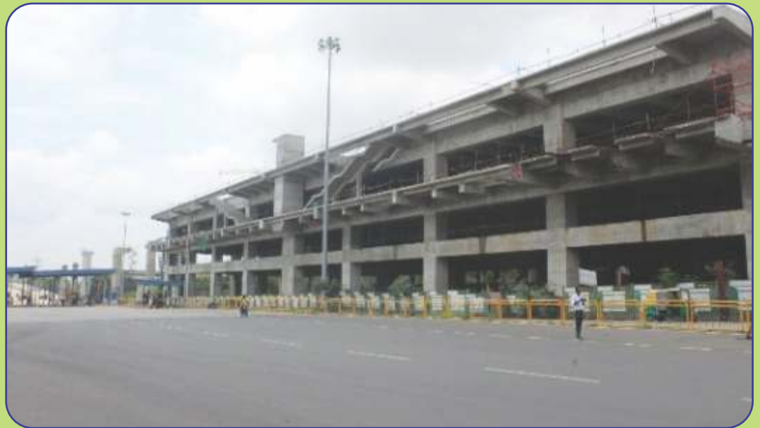
Electronic City Station works in progress - Reach 5
