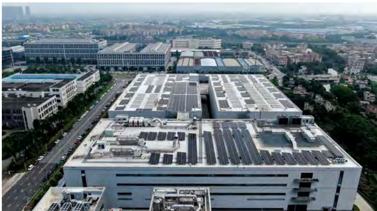
The array consists of roughly 38,000 individual solar panels – making it one of Freudenberg’s largest.
